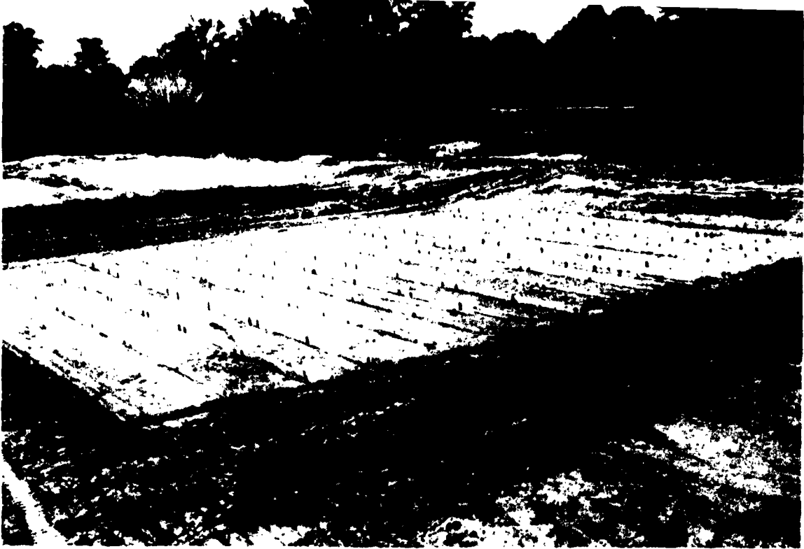
Fig. 4. Lean clay subgrade plot before topsoiling
