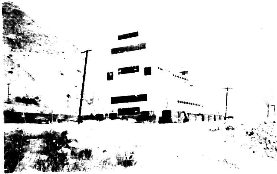
Figure 3. Looking west at steel-frame mill building. Explosion occurred at face of hill just left of upper part of building.
