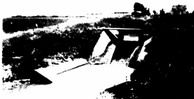
Photo 28. A single drop. These are located where there is a change of level of less than 5 feet. On aerial photos a drop appears only as a dark indistinct feature in the canal. Often drops are located where a change in level is associated with a change in direction. The stilling basin below the drop appears on aerial photos as a widening in the canal.
