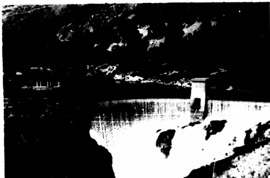
Photo 9. Diversion Dam. Water is diverted from Sun River at this dam into the North Side Canal System, supplying irrigation water for the Greenfields Irrigation District. Outlet is to the left.
