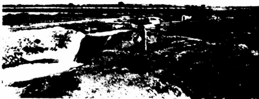
Photo 29. A series of drops. Note the stilling basins at the base of each drop.
