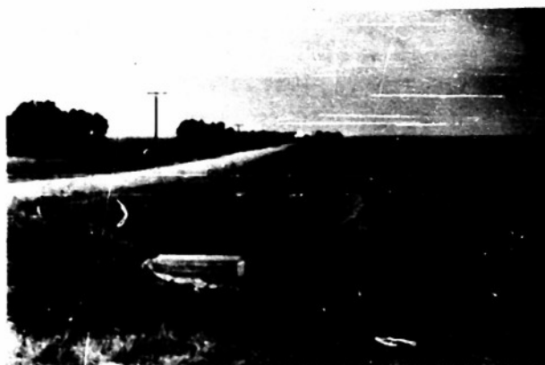
Photo 22. A head ditch along a highway. Note the turnoff into the border ditch. For aerial view of above ditch see (D) on Photo 19.
