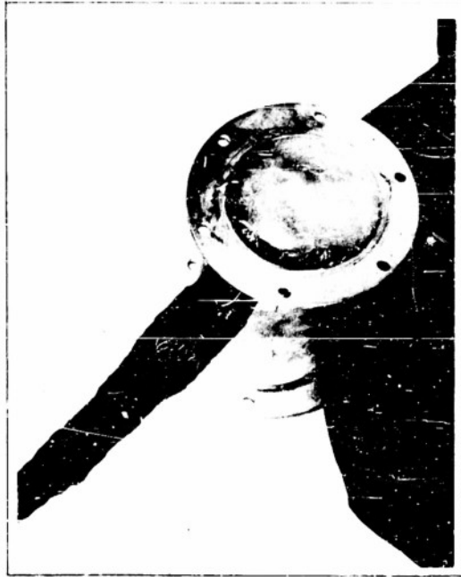
D. Fill connection chamber with silicone compound; wrap cable splice with friction tape
