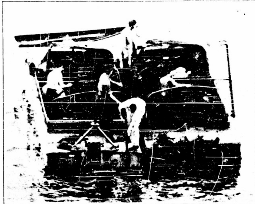
Fig. 21 — Installing cable at Pt. Arguello, California.
