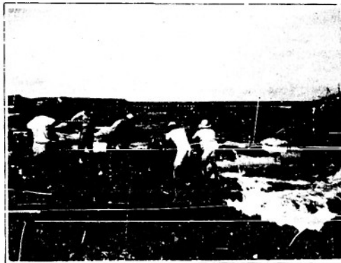
e. Electrical cable and chain being pulled off reef
