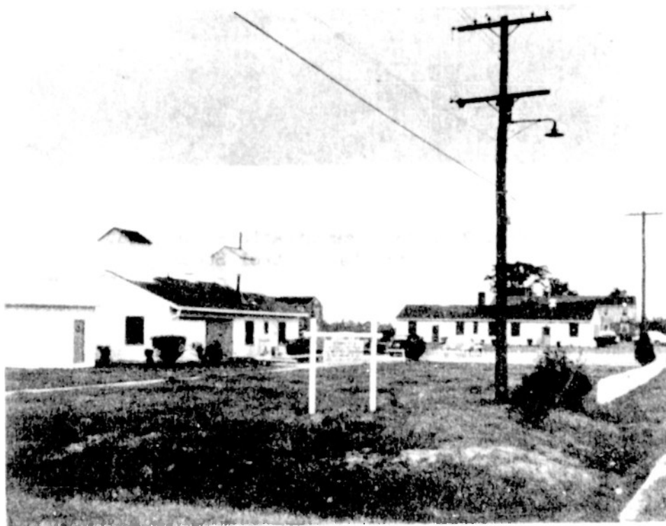
Fig. 2 Robins Project and Net Control building
