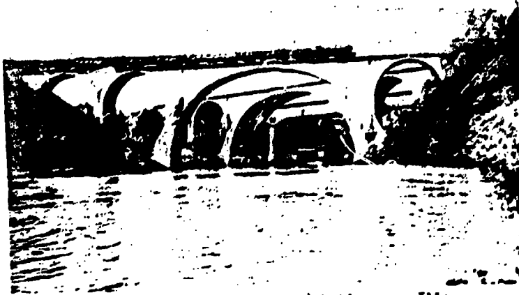
27. KEMPTEN (Route 118, 120) bridge over Iller.
