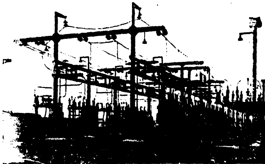
37. View of step-down side of open air installation of Freuchtlingen (Gronhart) sub-station, Augsburg-Auremberg electrified line.
