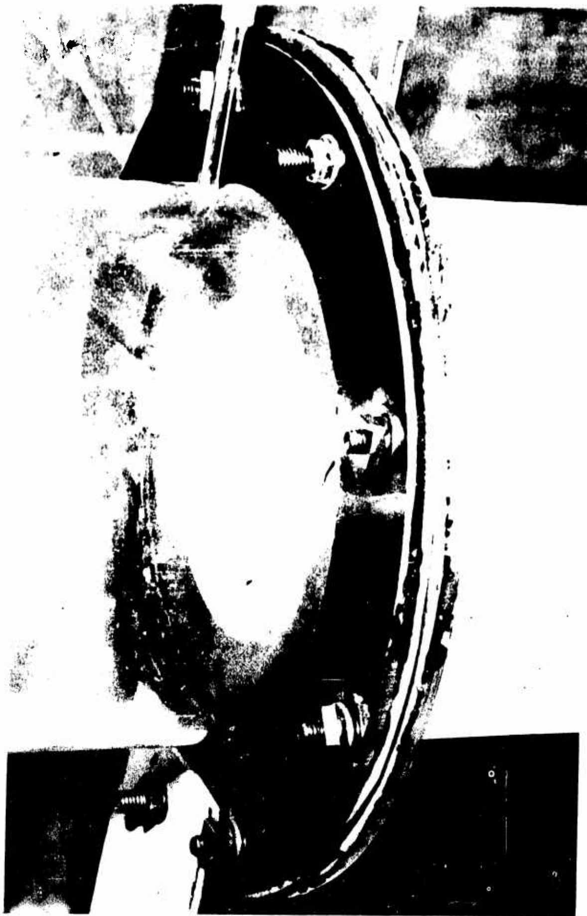
Figure 3. Typical Orifice Installation.
