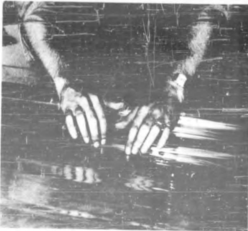
Figure III-20. The edge is folded back and tipped up until it "flips" down in place on the adhesive. At this point the seal is carefully inspected for wrinkles which may form air channels through the seal. Large bubbles trapped by the seam are individually run to an edge by finger pressure.
