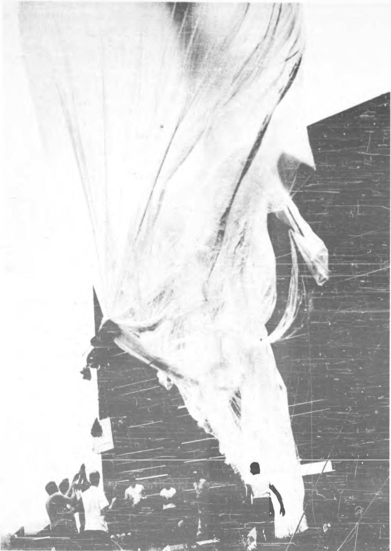
Figure II-11. The weight of the canopy shifting off center pulls the top of the bubble down.
