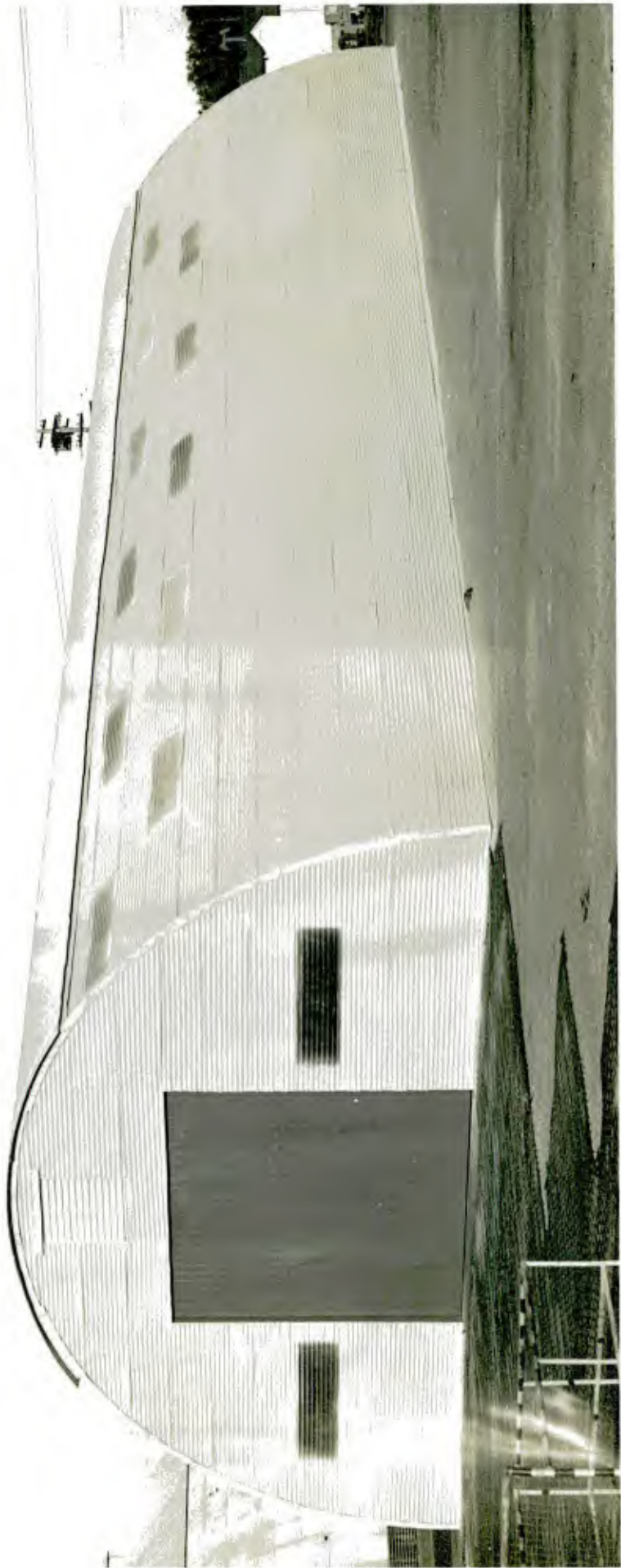
Figure 1. Standard Arch-Rib, 40-Ft by 100-Ft, Utility Building.
