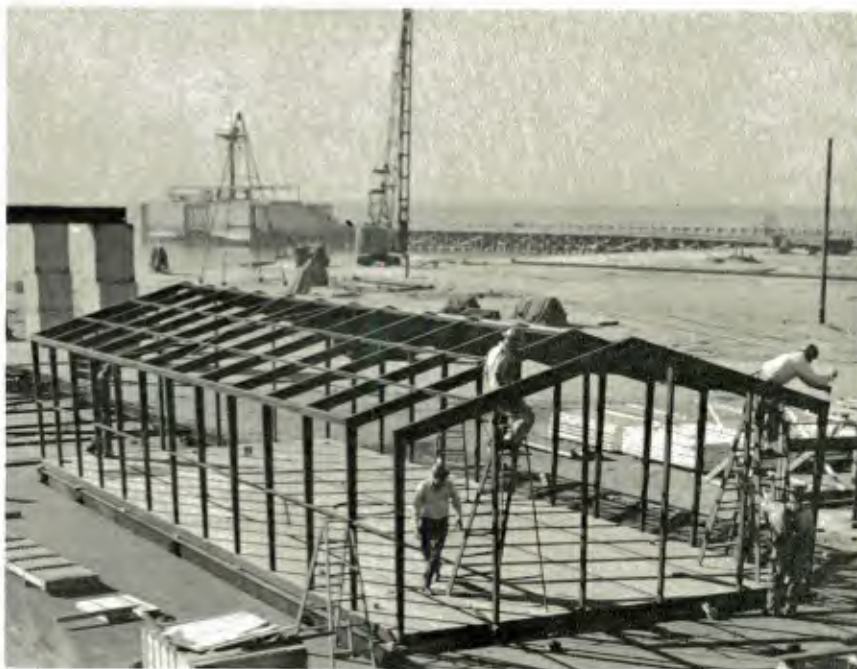
Figure 5. Structural frame of building.
