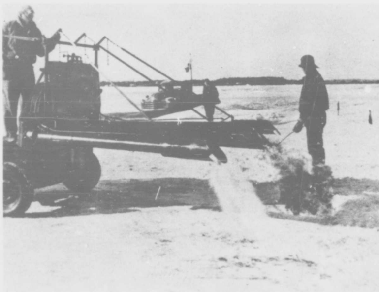
Figure 9. (Top) Woolery weed burner being towed by Harris tractor. (Bottom) Melting of icy surface with Woolery weed burner.
