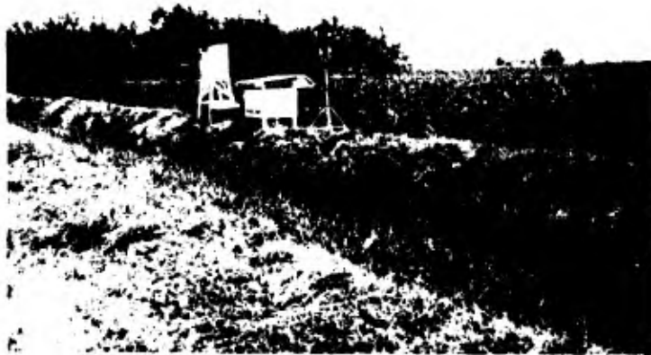
Figure 5. Substation No. 4, on the north side of a cotton field, University of Arizona Experimental Farm, 8th and E Streets
