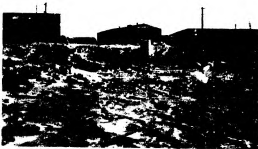
Figure 6. QM, South Camp Station. View looking east toward Corps of Engineers headquarters building.
