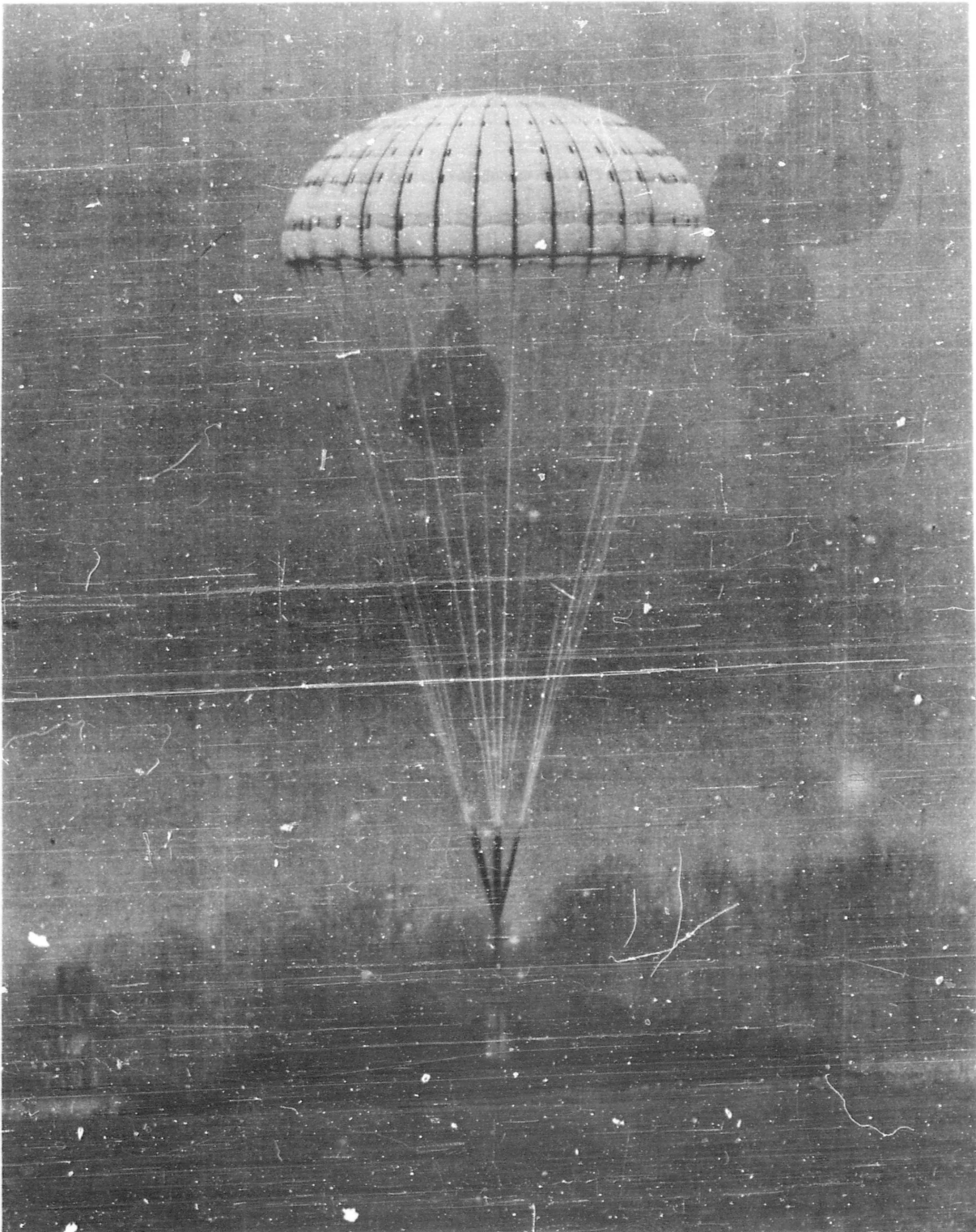
Figure 2.5.1 - Representative Photograph of a Fully Inflated Conical Ring Slot Canopy
