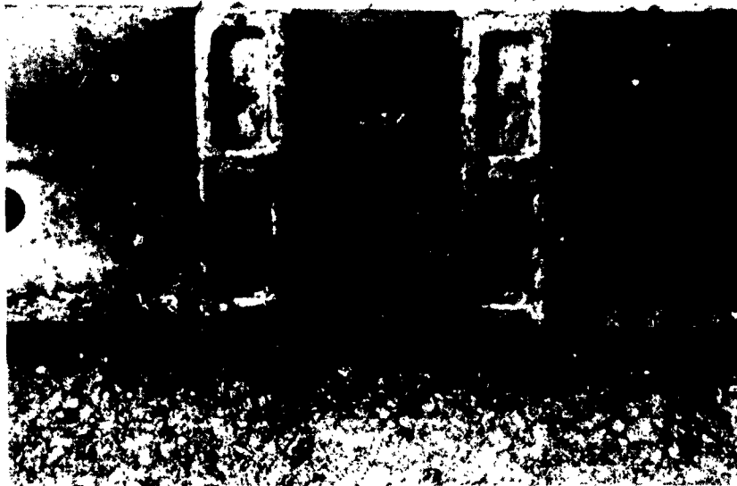
Figure 9. Rectangular link and pin holes located between the wedge bars on standard pontoon angle.
