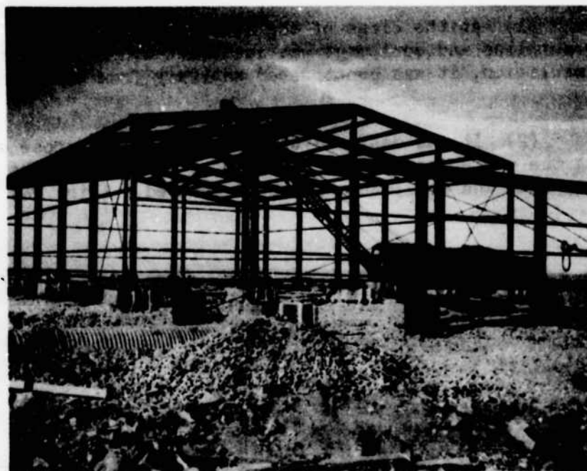
Fig. 22 Frame of Modular Building Erected for Mess Hall and Kitchen
