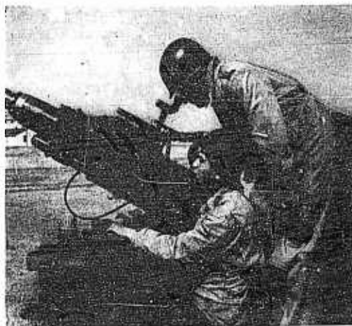
FIGURE 3. Elevation telescope bracket and elbow telescope M1A1 mounted on the M7 telescope on the elevation side of the gun. If a check on tracking during firing is desired, this arrangement is recommended.
