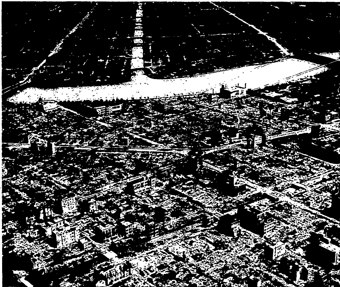
FIGURE 14. Nihonbashi District in Tokyo after attack of March 9, 1945, with AN-M69 incendiary bombs. The area in this picture is within one mile of the area shown in Figure 13 and has the same type of construction. Note the gutted shells of modern concrete buildings and complete destruction of the Japanese type buildings ( Life photograph).
