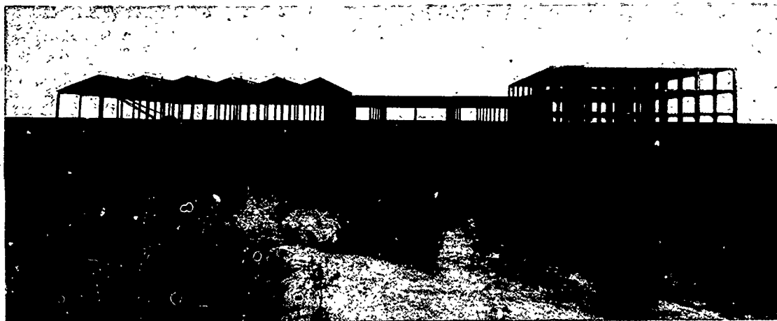
FIGURE 28. View of an Eglin Field factory-type, incendiary test building.
