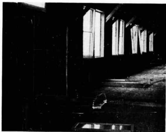
FIGURE 40. Barracks damage, Test 1.
