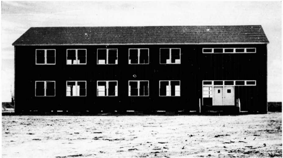
FIGURE 29. Barracks damage, Test 1. West elevation (exposed to blast).
