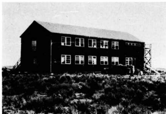
FIGURE 5. Navy-type barracks building.
