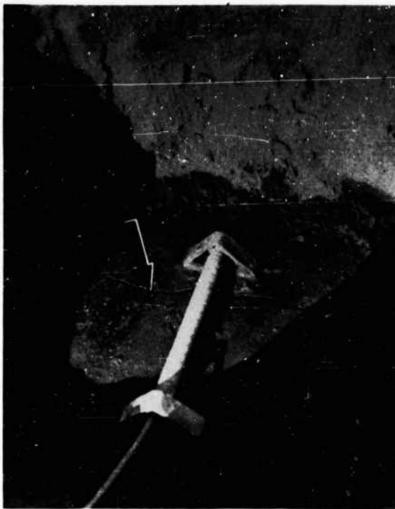
FIGURE 72b. Carlson Strain Meter No. 2 installed showing crack.
