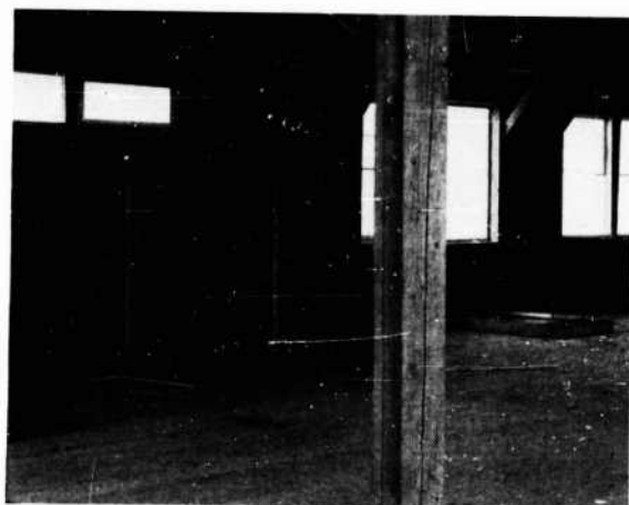
FIGURE 39. Barracks damage, Test 1.
