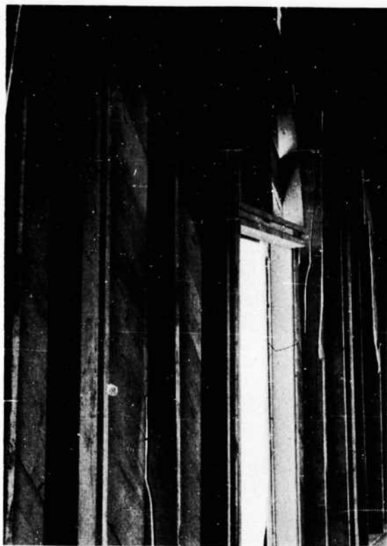
FIGURE 35. Barracks damage, Test 1.
