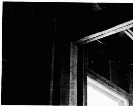
FIGURE 41. Barracks damage, Test 1.
