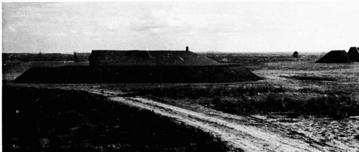
FIGURE 64. Revetment 1, Igloo C, and (right) door barricade at Igloo B, prior to Test 2.
