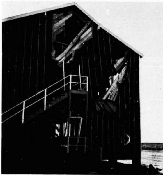
FIGURE 80. Barracks damage, Test 3.
