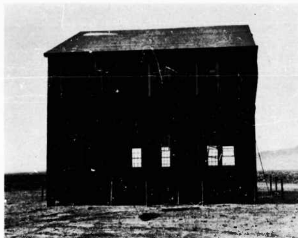
FIGURE 55. East elevation of Barracks 1 after Test 1
