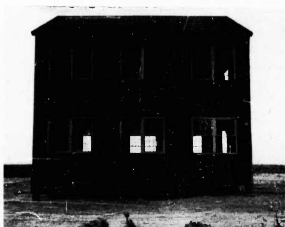
FIGURE 156. East elevation of Barracks 2 after Test 3
