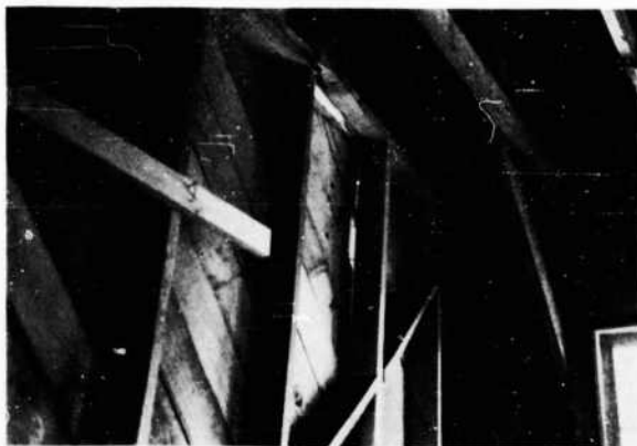
FIGURE 72. Interior, Barracks 2 after Test 1. Second story, northeast corner, showing broken plate and displaced stud
