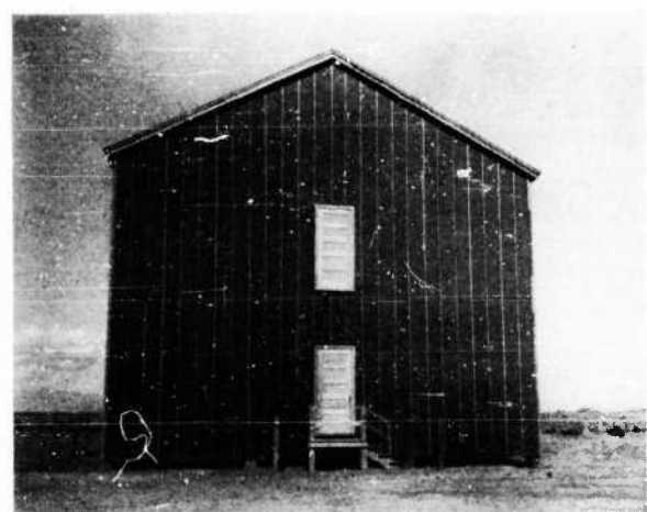
FIGURE 57. South elevation of Barracks 1 after Test 1
