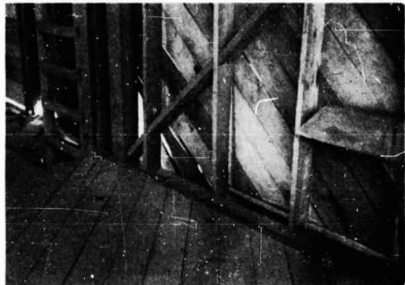
FIGURE 166. Interior, Barracks 1 after Test 3, illustrating displacement of south wall at second floor level
