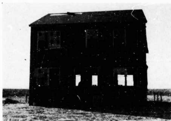
FIGURE 108. East elevation of Barracks 1 after Test 2
