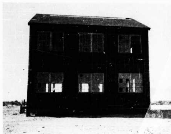
FIGURE 213. East elevation of Barracks 3 after Test 5
