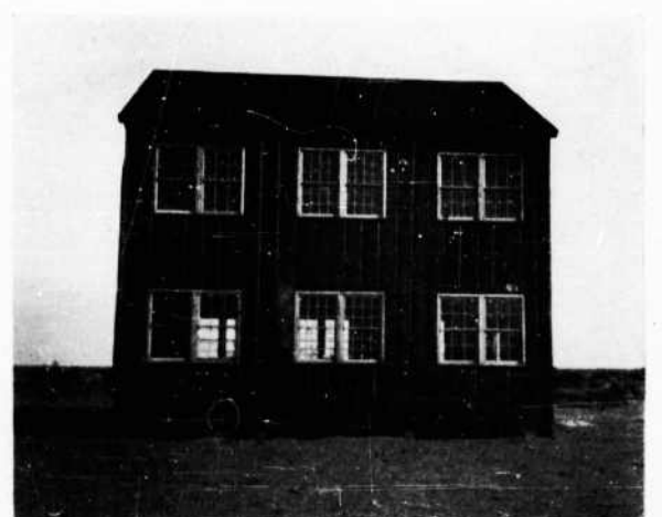
FIGURE 162. West elevation of Barracks 3 after Test 3
