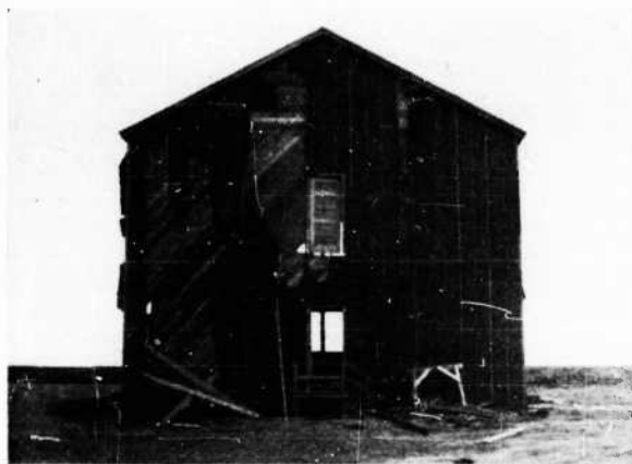
FIGURE 185. Barracks 1 after Test 4; south elevation
