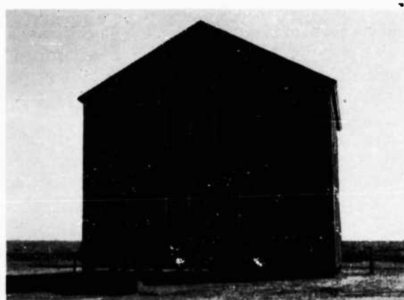
FIGURE 110. North elevation of Barracks 2 after Test 2
