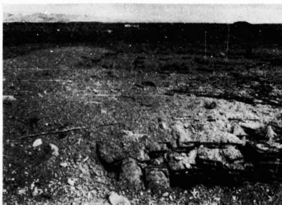
FIGURE 181. Revetment 2 after Test 4, looking north from south windrow
