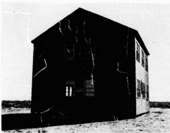
FIGURE 212. North elevation of Barracks 3 after Test 5
