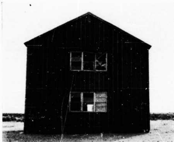
FIGURE 159. North elevation of Barracks 3 after Test 3
