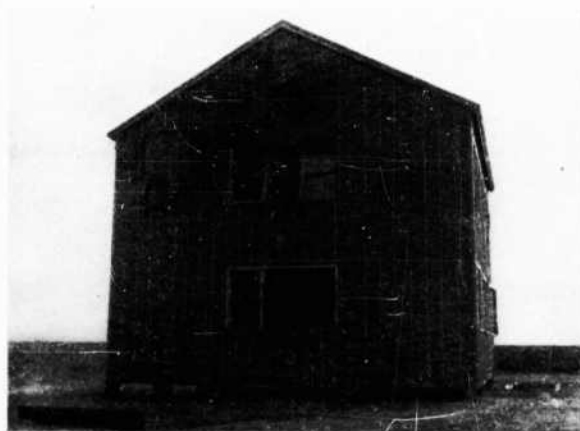
FIGURE 187. Barracks 2 after Test 4; north elevation
