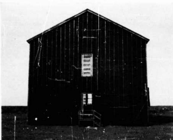
FIGURE 161. South elevation of Barracks 3 after Test 3
