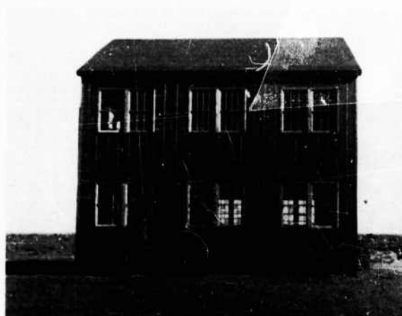
FIGURE 215. West elevation of Barracks 3 after Test 5
