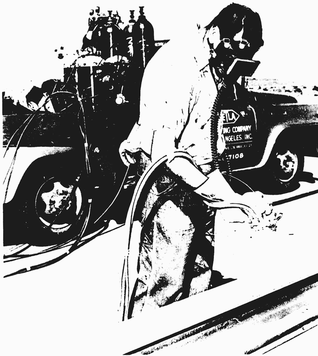
FIGURE 8. Six Percent Antimonial Lead Metallizing Operation
