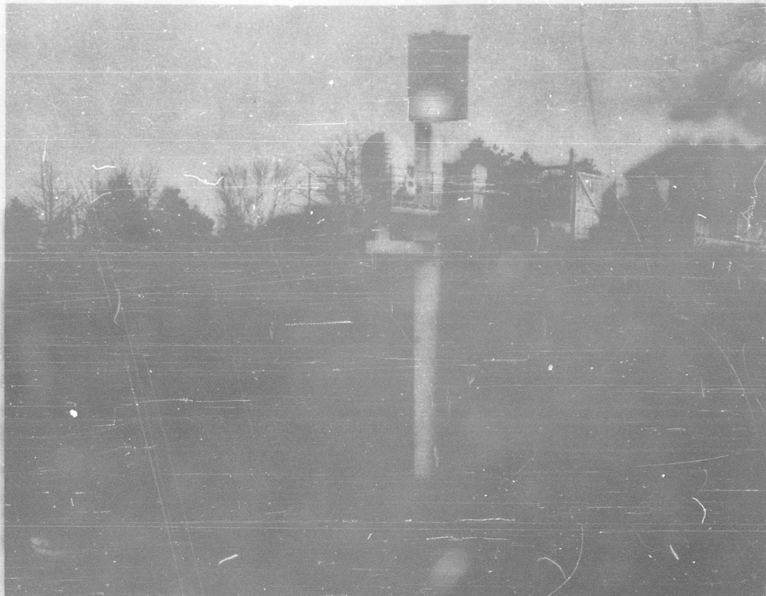
Fig. 5 - Drop-test structure installations
