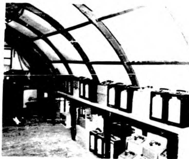
FIGURE 7: ARRANGEMENT OF RECORDING INSTRUMENTS IN JAMESWAY SHELTER.
