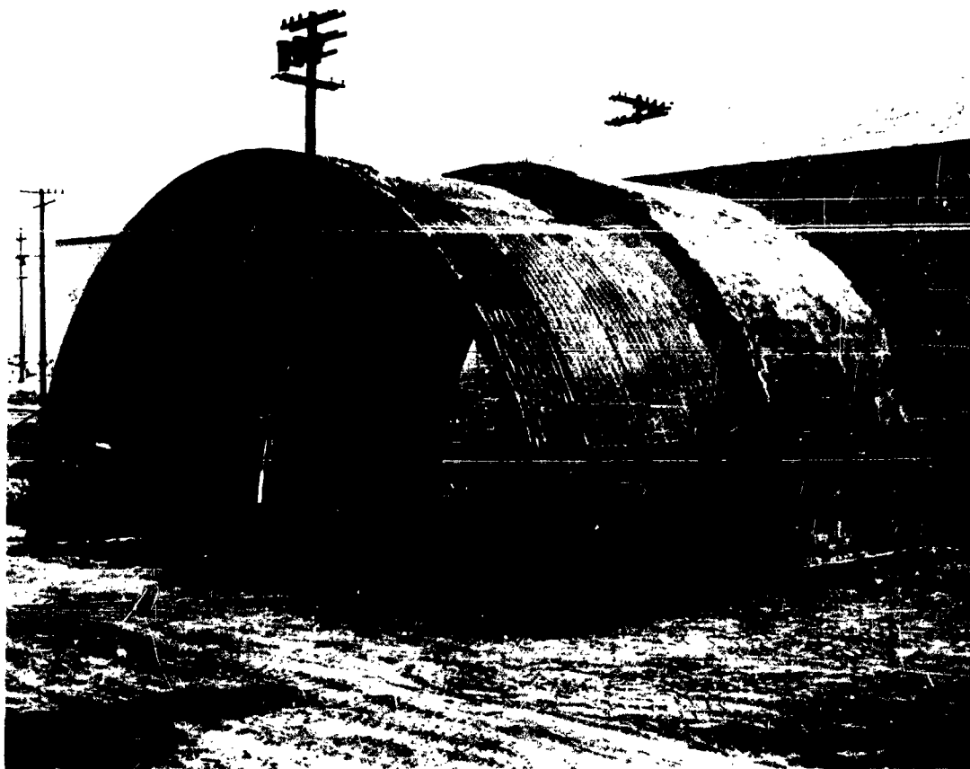
Figure 3. Quonset form and shotcrete arch.
