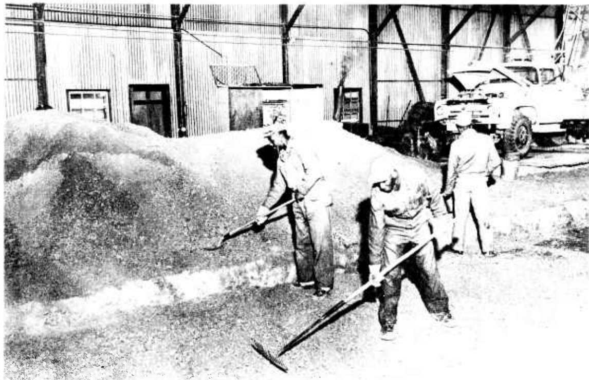
a. Placing a lift of soil
