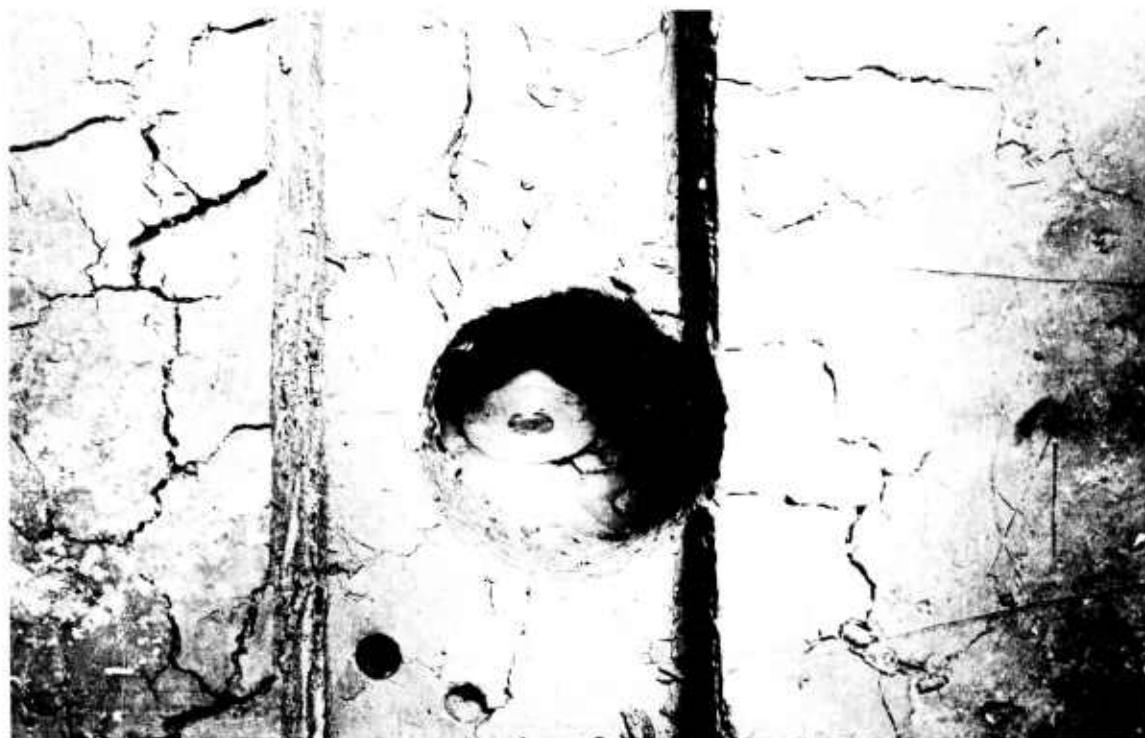
Fig. 13. Uncovered cell CEC 639 (at sta 0+60) after completion of test 2
