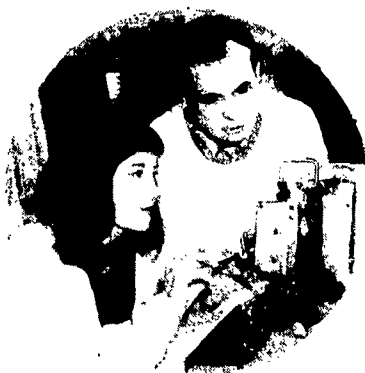
Upper (center) illustration: Technician N. K. Saricheva together with co-worker of the Experimental Medicinal Laboratory im. October Revolution V. I. Babich assemble a device (bath) for examining tissues and human organs with the aid of ultrasonic oscillations.
