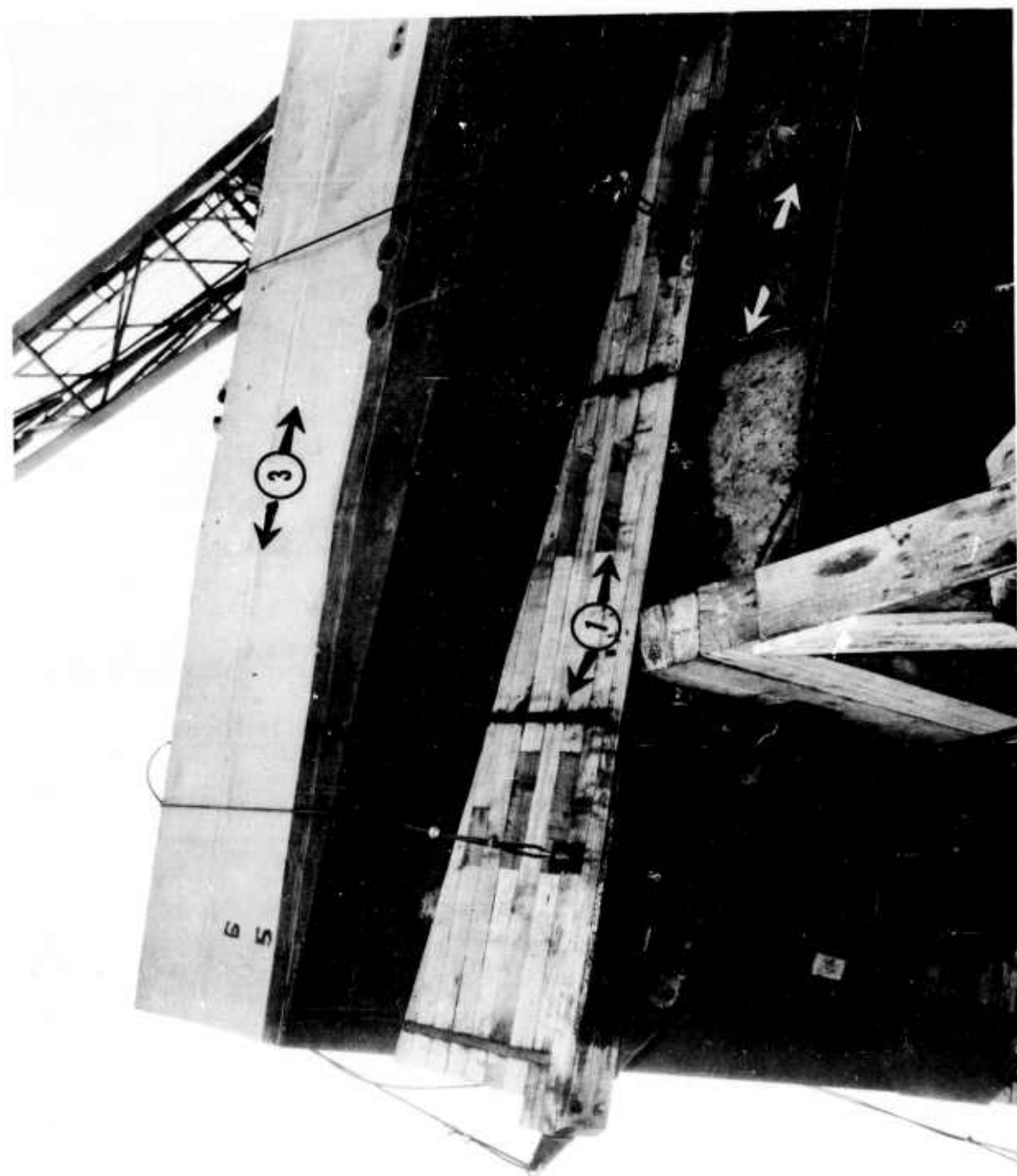
Figure 14. The LCM-8 and the Sliding Ways Mounted on the Ground Ways. Note sliding ways (1), ground ways (2), and the position of the tracing lines (3).
