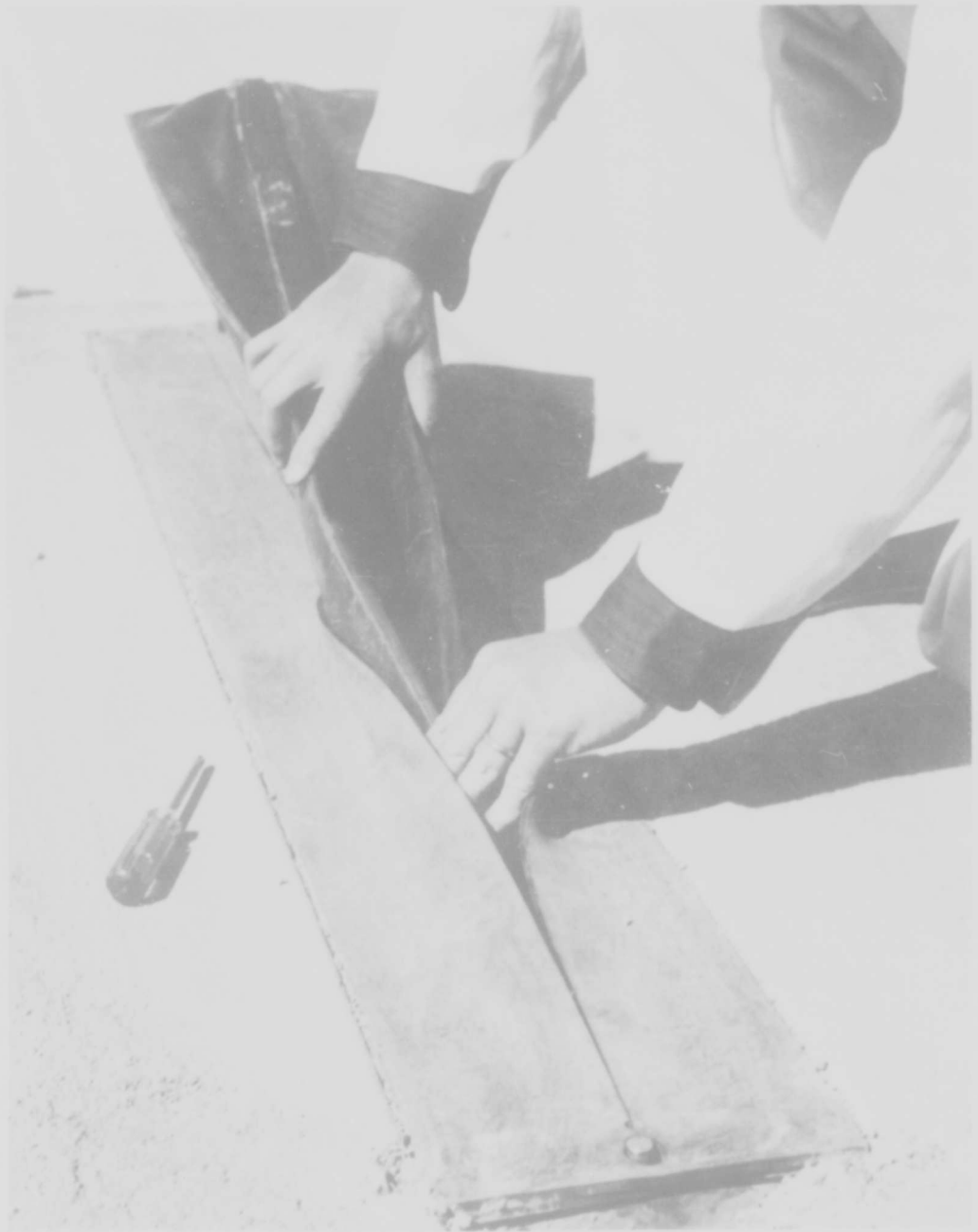
FIGURE 33: INSTALLING TROUGH UNIT AIR BAG
