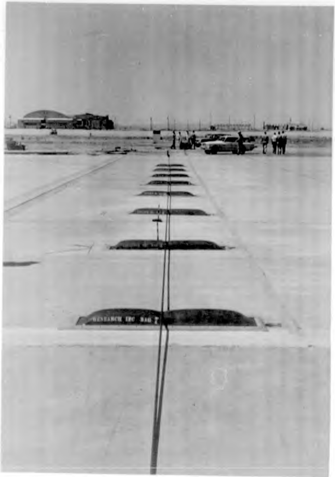
FIGURE 21: INFLATABLE CABLE SUPPORT INSTALLATION
