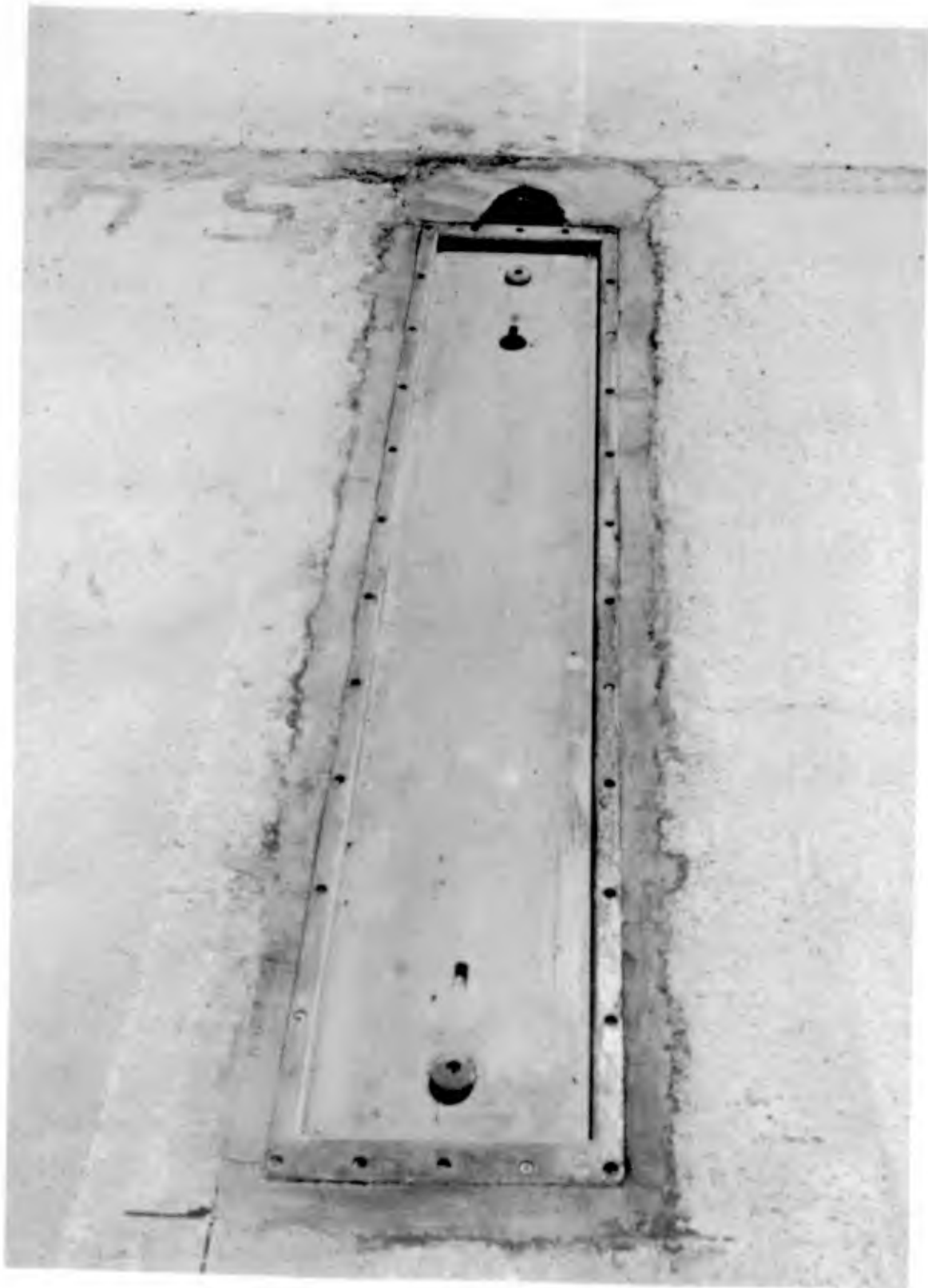
FIGURE 10: FLUSH MOUNTING BASE INSTALLATION
