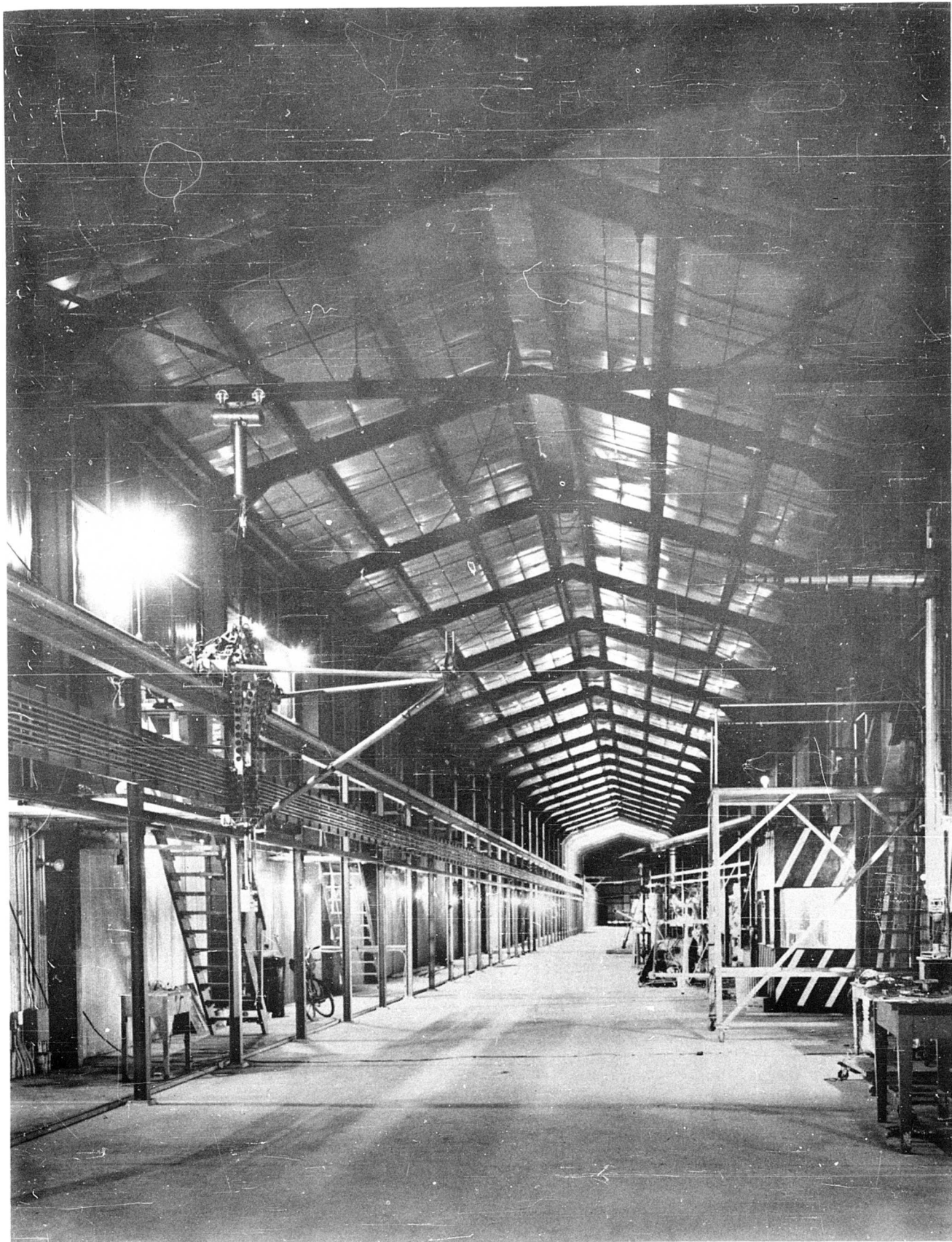
Figure 1 INTERIOR OF TRACK
