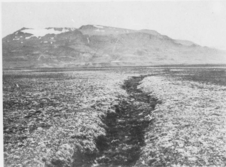
Photograph 13. Frost crack that crosses center of surveyed runway site at Storely.
