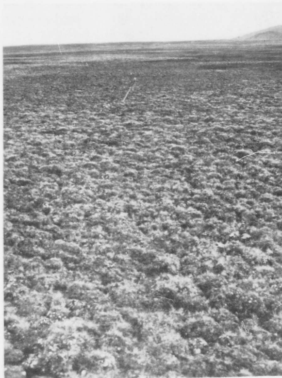
Photograph 12. Typical surface near center of 11,500-foot runway site near Storelv, showing typical size of hummocks that occur from 4000 to about 6500 feet from the northwest end of the strip. Typical dimensions of the hummocks shown are 6 to 12 inches in diameter and 2 to 6 inches high. Hummocks of this size would probably permit safe landings and takeoffs by planes of the C-130 type. View is S15° E, along the center-line, near its midpoint. Date: 1 September 1959.
