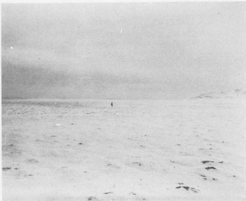
Photograph 14. View along the surveyed runway at Storely after snowfall. View is from the northwest corner, looking southeast. The flag in the foreground marks the corner of the strip, which is 200 feet wide. The centerline extends into the background and to the right, marked by flags spaced 500 feet apart, at least two of which are visible near the corner-marker. Date: 5 September 1959.
