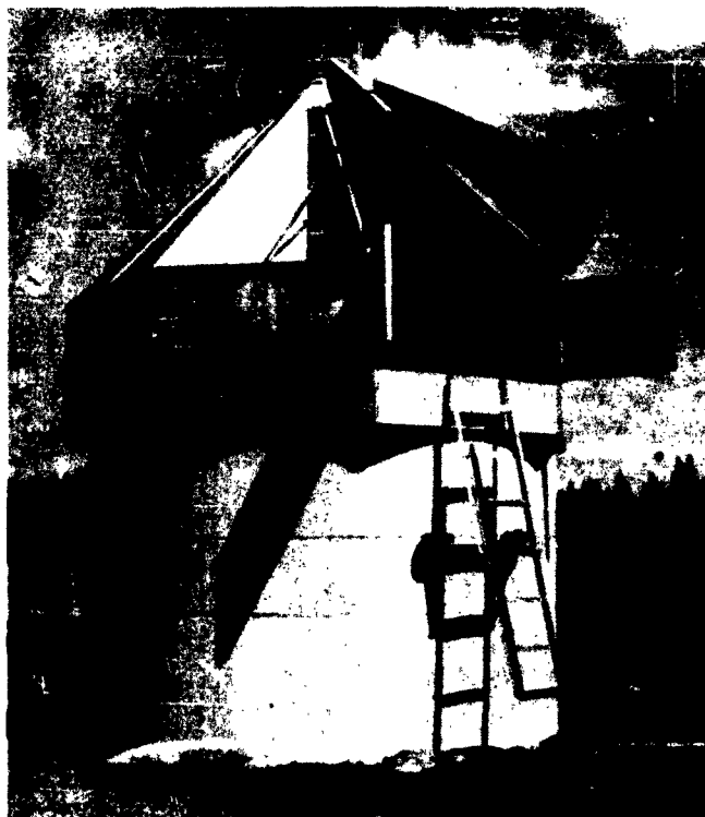
Fig. 1. Small observatory housing the Zeiss Coudé telescope of the Oslo Solar Observatory. The whole top of the construction turns to follow the sun.
