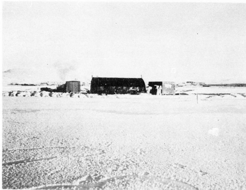
FIG. 4.8. Surface of Parking Apron No. 1 after completion (official photograph, U. S. Navy)
