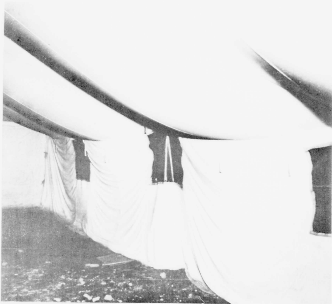
Figure 7. Tent, Interior, Showing Sagging of Liner
