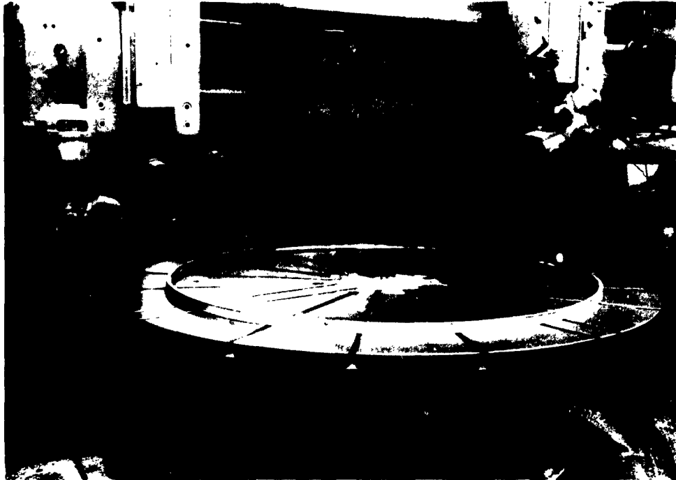
Fig. A-5 Frame Ready for Turning
