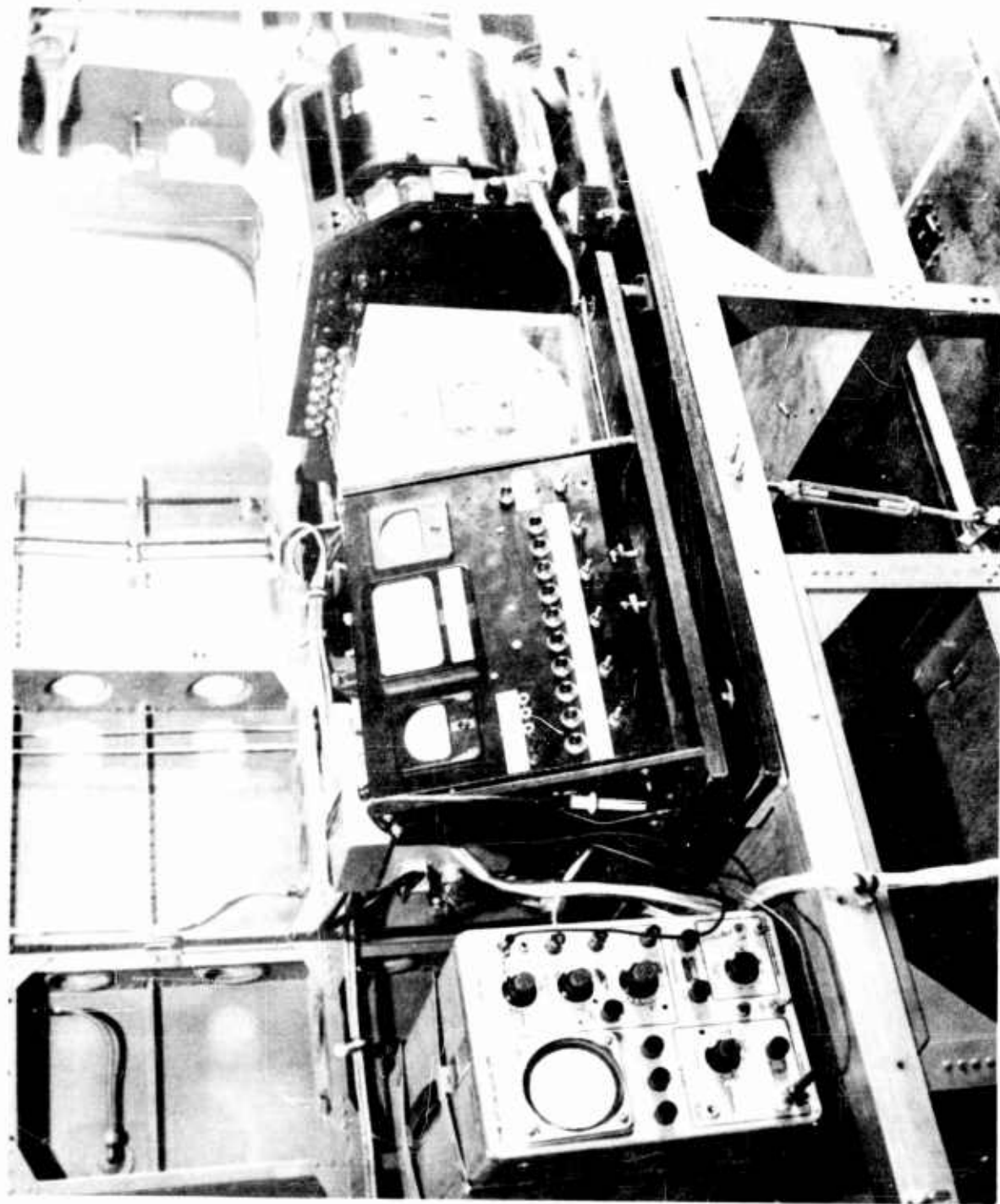
Figure 20. System Equipment Installation, H-37.
