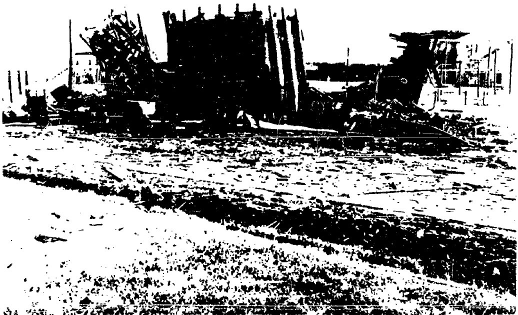
Slide 1 Explosion - Propellant Blending Building
