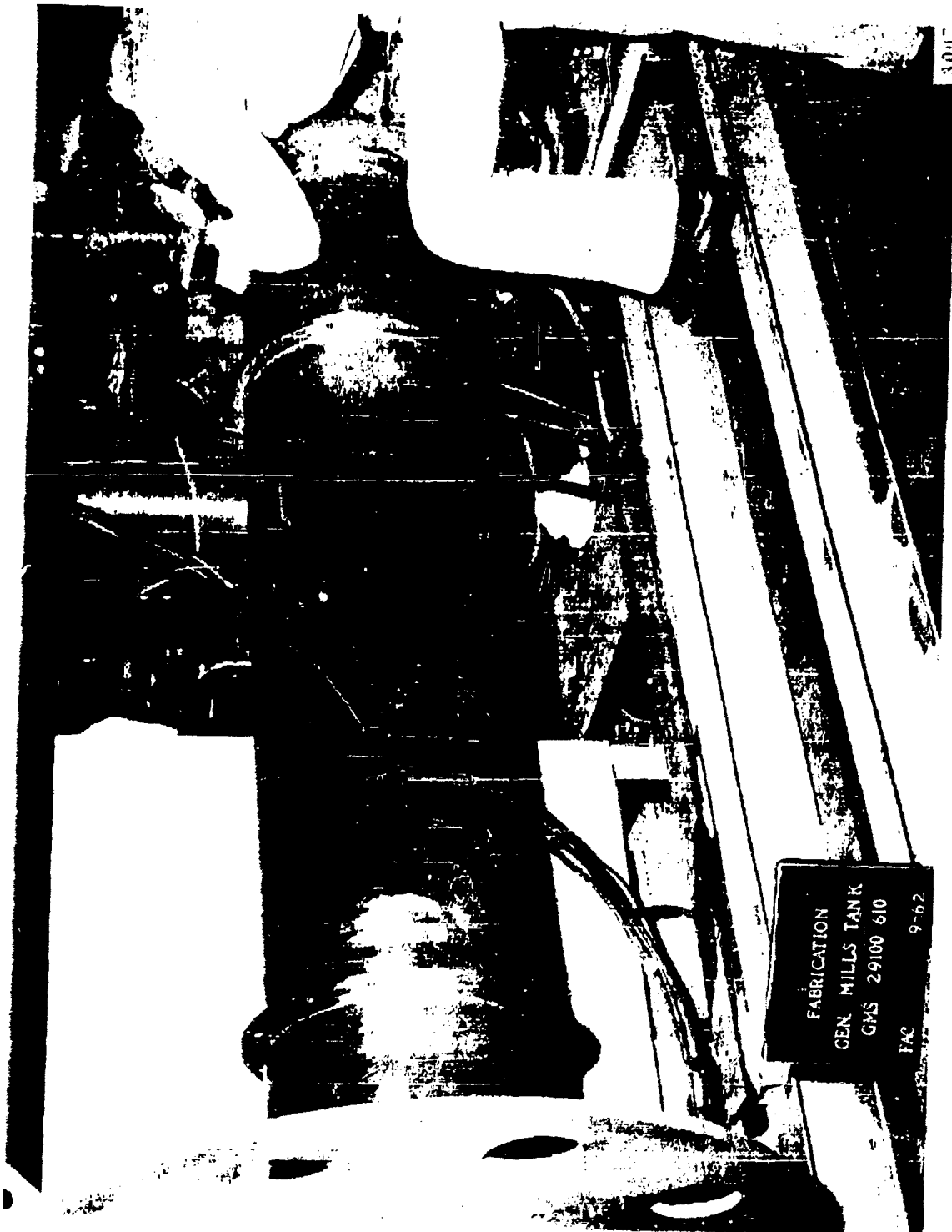
Figure 6.4 Welding an End Ring on Inner Tank
