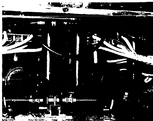
Figure 5 - HPA configuration, bottom side. The 3-1/8-in. coaxial lines contain the grid shunt tuners. The water hoses and filament-supply leads are nearly the same size. Resistors at the bottom are for parasitic suppression.
