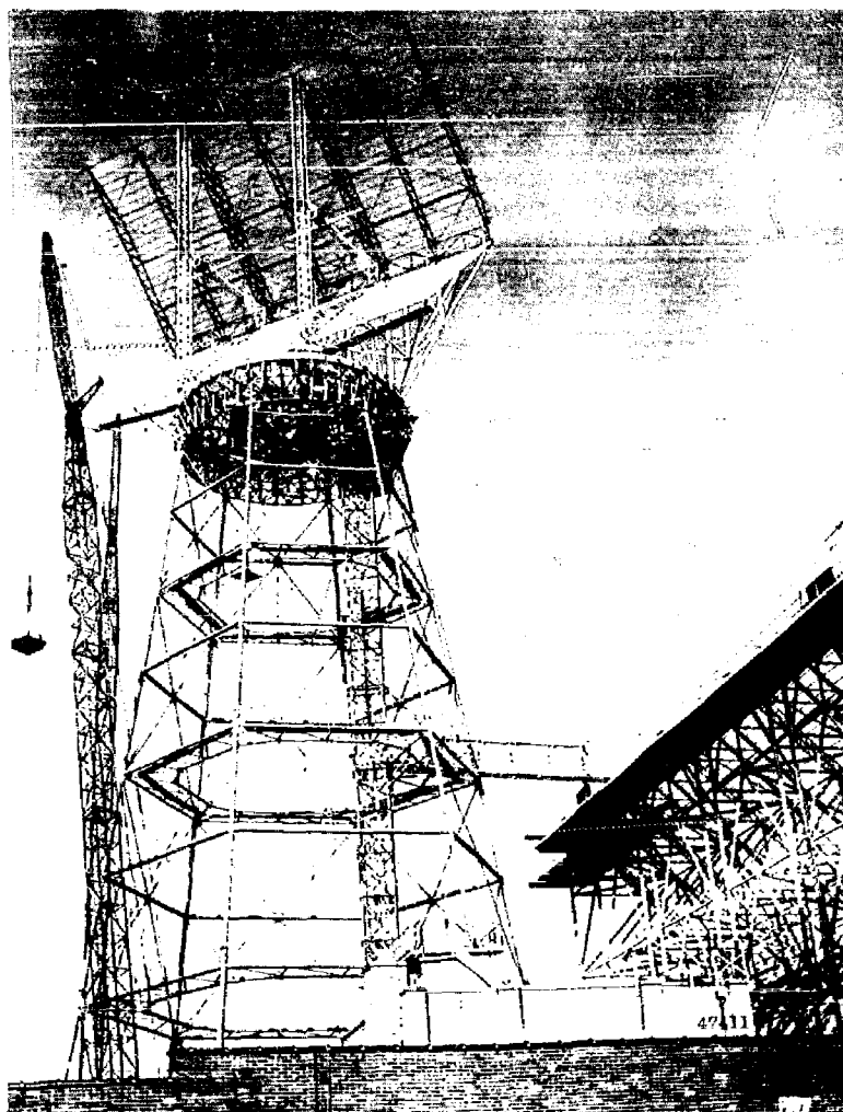
Figure 26 - Positionable antenna. The elevator shaft and catwalk are visible. To the right, a portion of the rear of the fixed antenna is visible, showing the concrete loading weights.
