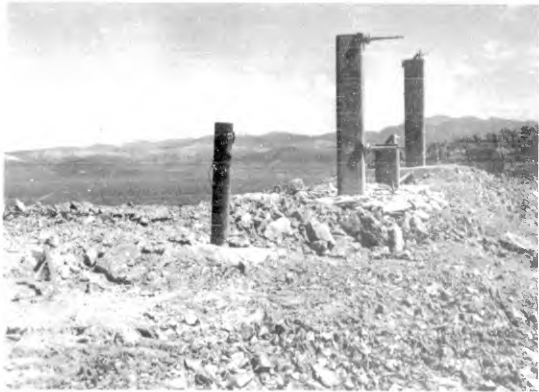
Figure 3.4 Typical gage installation, top of ridge.
