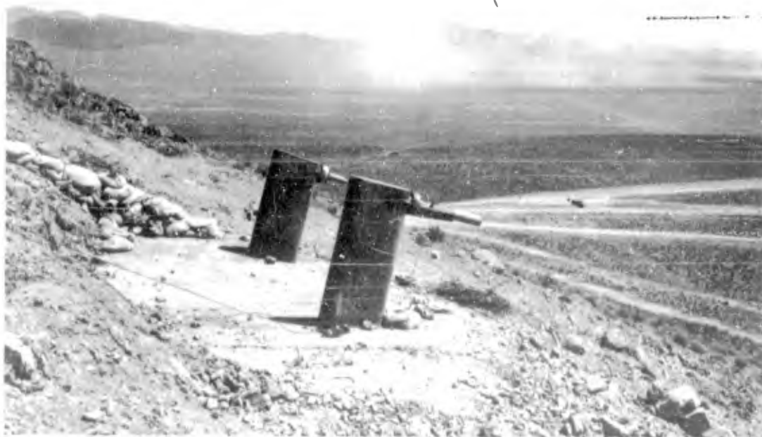
Figure 3.3 Typical gage installation, front slope.
