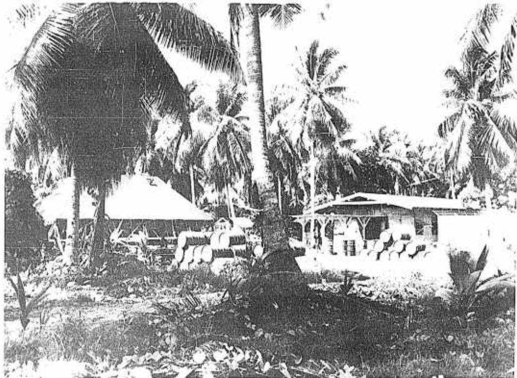
Figure 2.3 General view of maintenance facilities of Project 4.1, on Site David, Eniwetok Atoll. Tent in the left foreground housed up to 670 rabbits. Building at the right housed up to 48 monkeys, the shutter and electronic test and assembly laboratory, and a semi-darkened ocular examining room.
