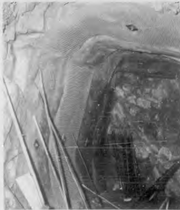
Figure 2.25 Rock bolt installation, square test section. (H&N-AEC 60-779-7, 1960).
