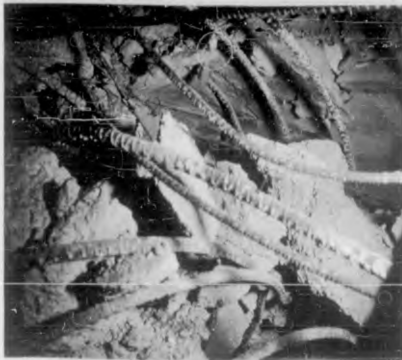
Figure 3.62 Close-up, west half B3b at 45° (post-shot). Note exposed polyurethane foam behind reinforcing bars (DASA - NOU 237-12 NTS-62)
