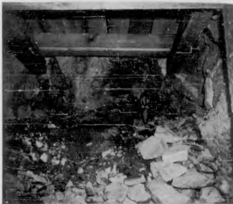
Figure 3.23 Access tunnel from Sta 5+00, approximately 310 feet from zero point, view to north (post-shot) (DASA - NOU 377-01 NTS-62).
