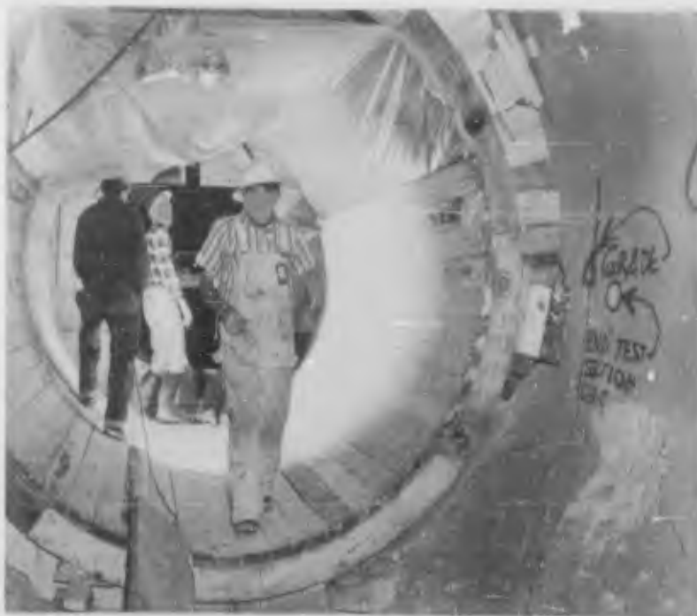
Figure 2.15 Installing tongue-and-groove forms for polyurethane foam. (H&N-AEC 789-1, 1960).
