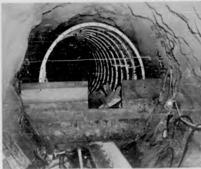
Figure 2.6 End bulkhead for corrugated steel tunnel liner partially installed. (LRL Photo, 1960).
