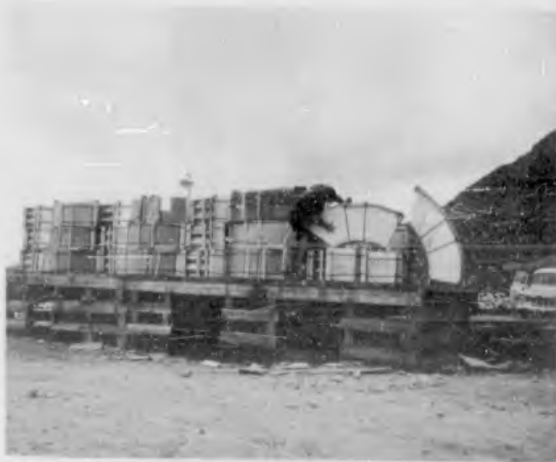
Figure 2.34 Preformed tunnel liner plates, as delivered to site (DASA - NOU 037-10 NTS-62).
