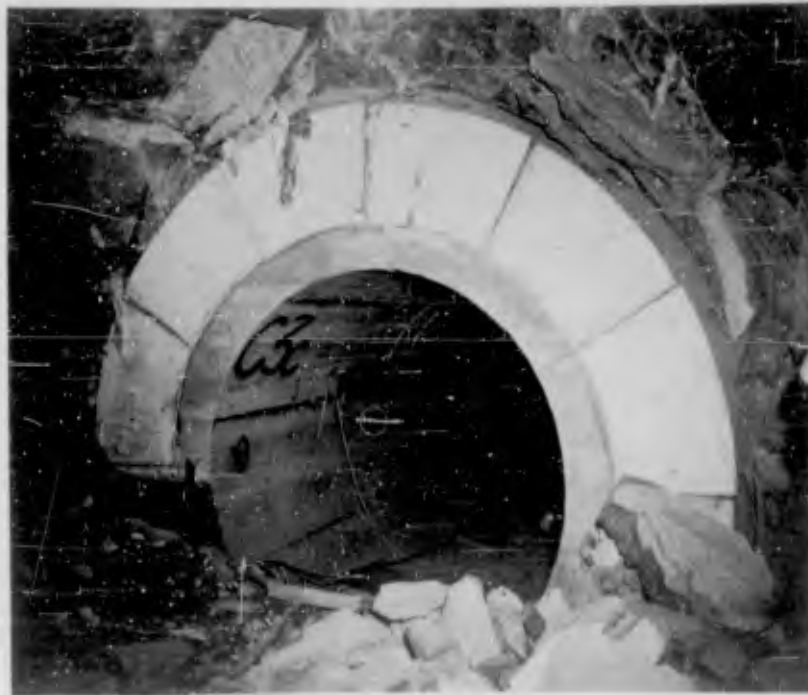
Figure 3.24 Test Section C3c (postshot) (DASA - NOU 339-09 NTS-62).
