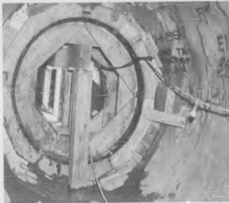
Figure 2.21 Concrete liner, forms installed. (H&N-AEC 789-2, 1960).
