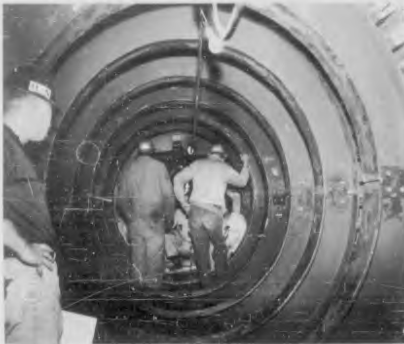
Figure 2.29 Wide flange rings installed, ready for welding (DASA - NOU 043-10 NTS-62).
