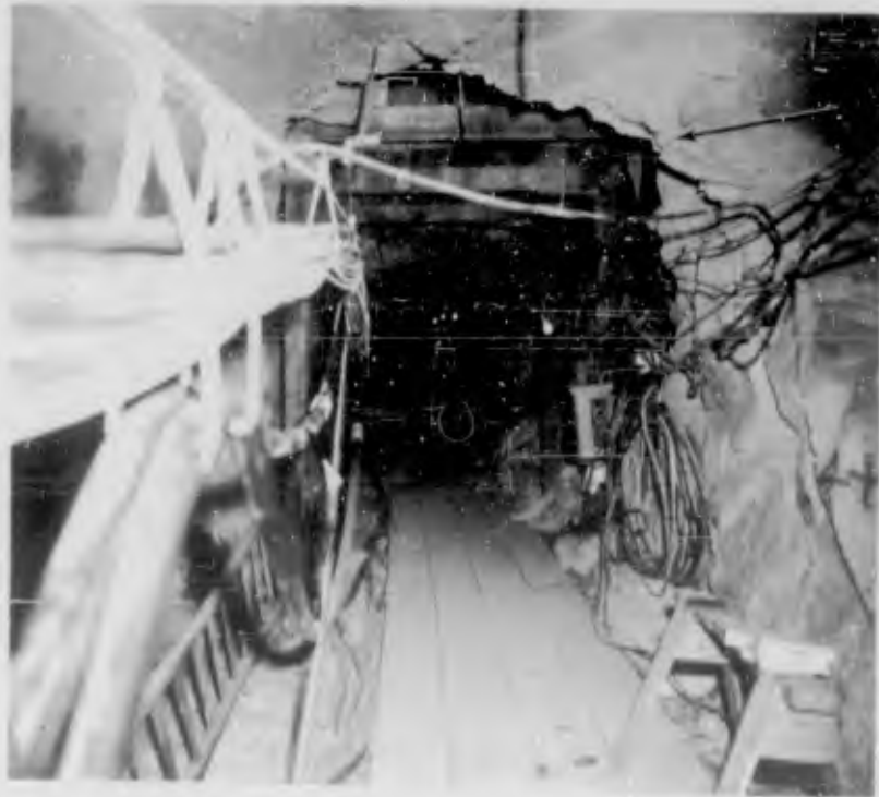
Figure 3.20 Access tunnel from Sta 4+75, approximately 335 feet from zero point, view to north (pre-shot). Note timber sets (DASA - NOU 085-01 NTS-62).
