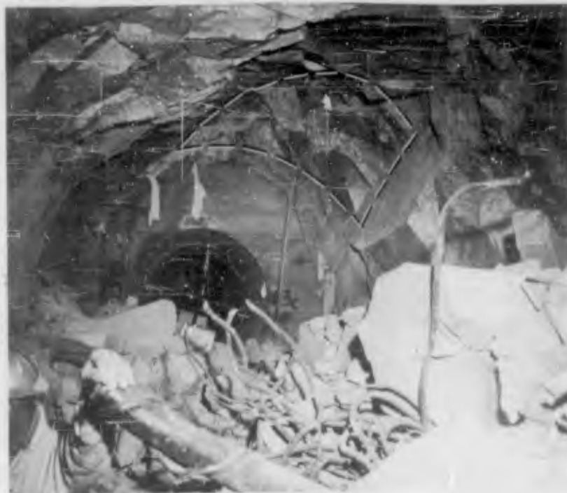
Figure 3.25 Transition zone, C Drift left. Note approximate rock breakage bounded by dotted lines (DASA - NOU 208-04 NTS-62).
