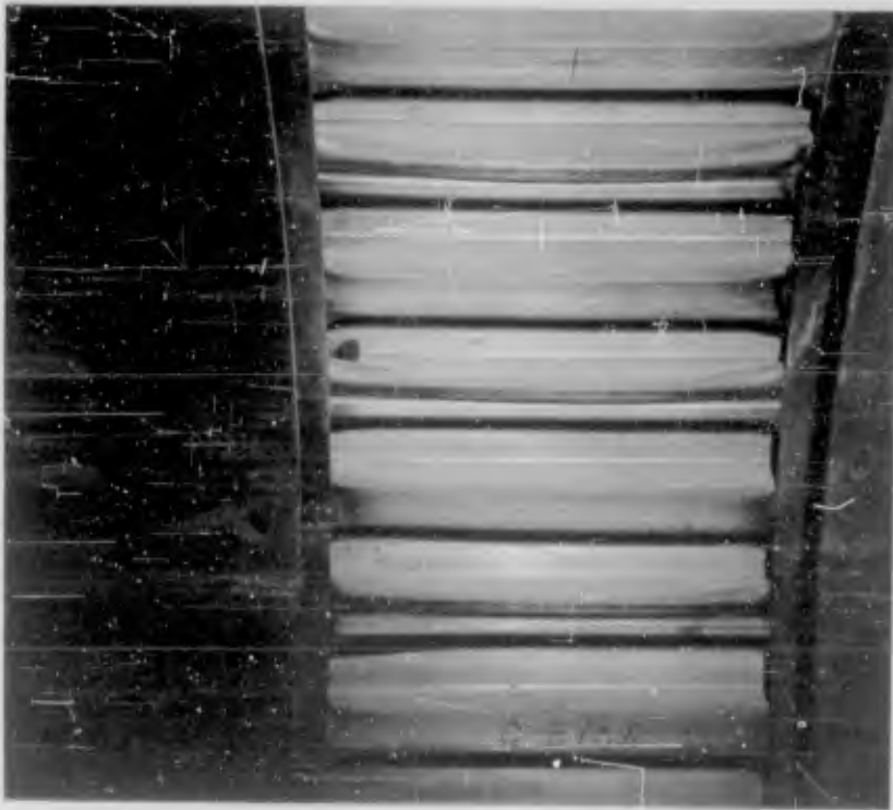
Figure 3.34 Close-up C4b. Note distorted steel decking (DASA - NOU 228-01 NTS-62).
