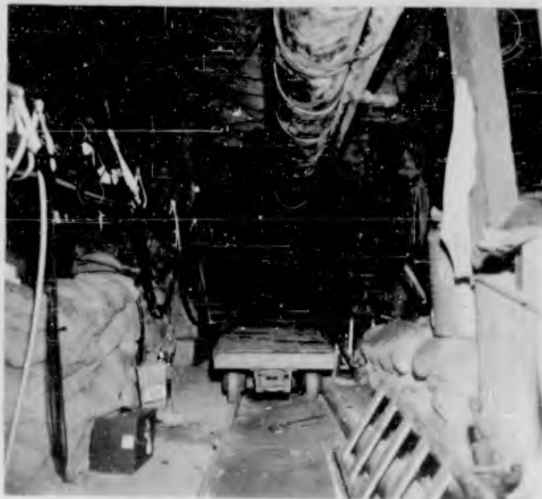
Figure 3.14 Access tunnel from Sta 3+00, approximately 505 feet from zero point, view to north (pre-shot) (DASA - NOU 085-09 NTS-62).
