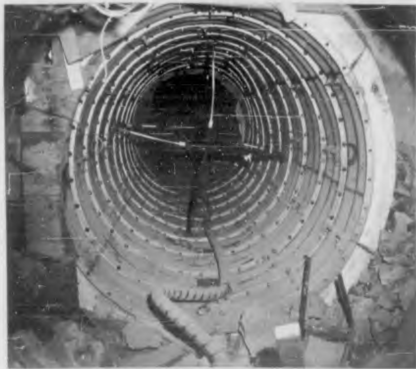
Figure 3.35 Test Section C6b (postshot) (DASA - NOU 227-12 NTS-62).
