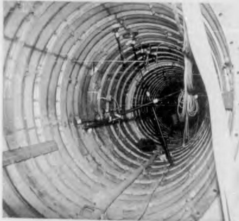
Figure 3.81 Interior view B5a (pre-shot) (DASA - NOU 073-11 NTS-62).
