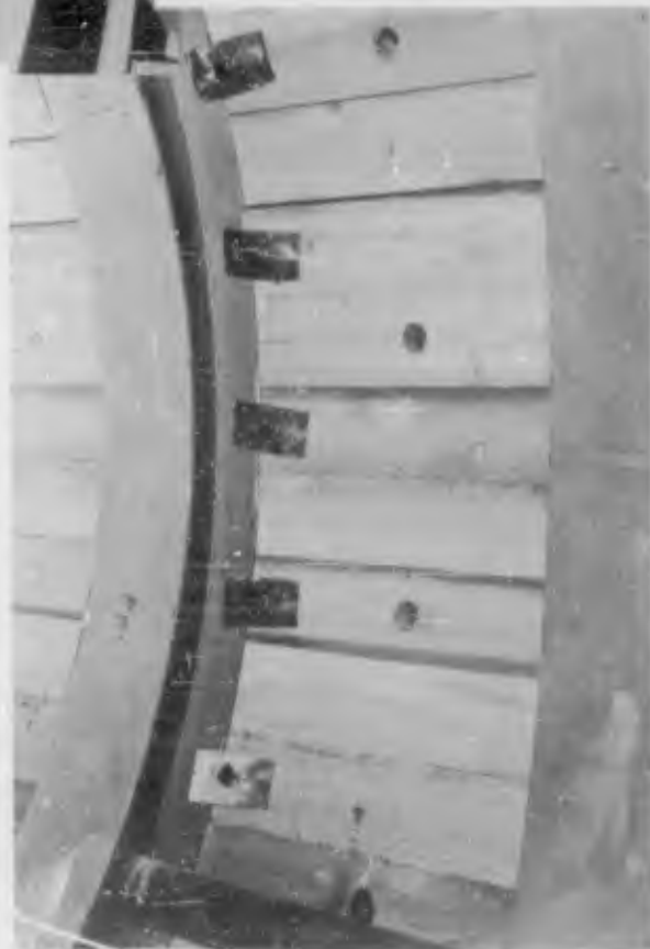
Figure 2.13 Details, wide-flange rings with wood lagging. (H&N-AEC 805A-2, 1960).
