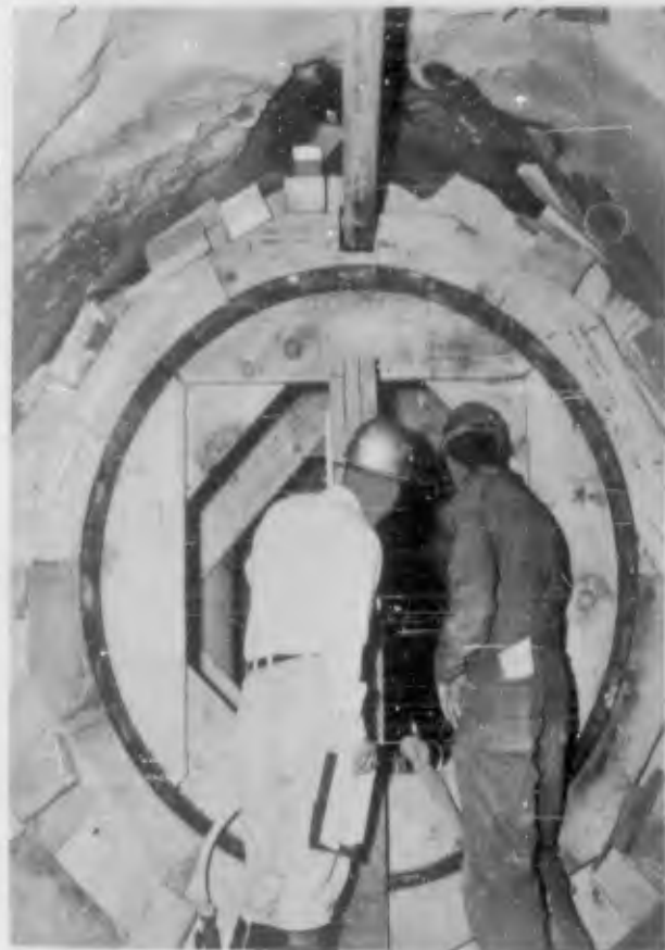
Figure 2.17 Typical concrete form construction. (H&N-AEC 789-8, 1960).
