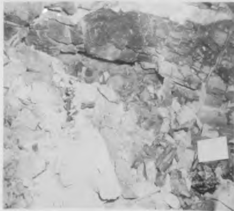
Figure 3.19 Access tunnel from Sta 4+00, approximately 410 feet from zero point, view to north (post-shot) (DASA - NOU 208-05 NTS-62).
