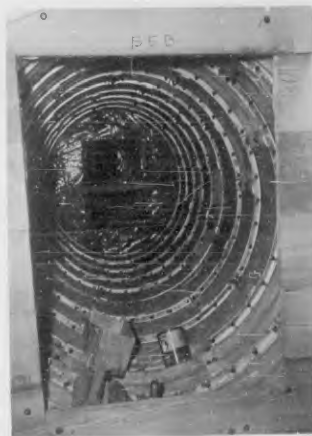
Figure 2.7 Corrugated steel tunnel liner completed. (LRL Photo, 1960).
