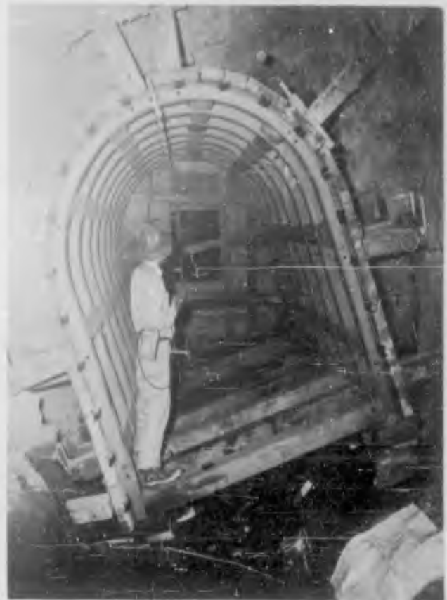
Figure 2.23 Steel horse- shoe sets with wood lagging. (LRL Photo, 1960).
