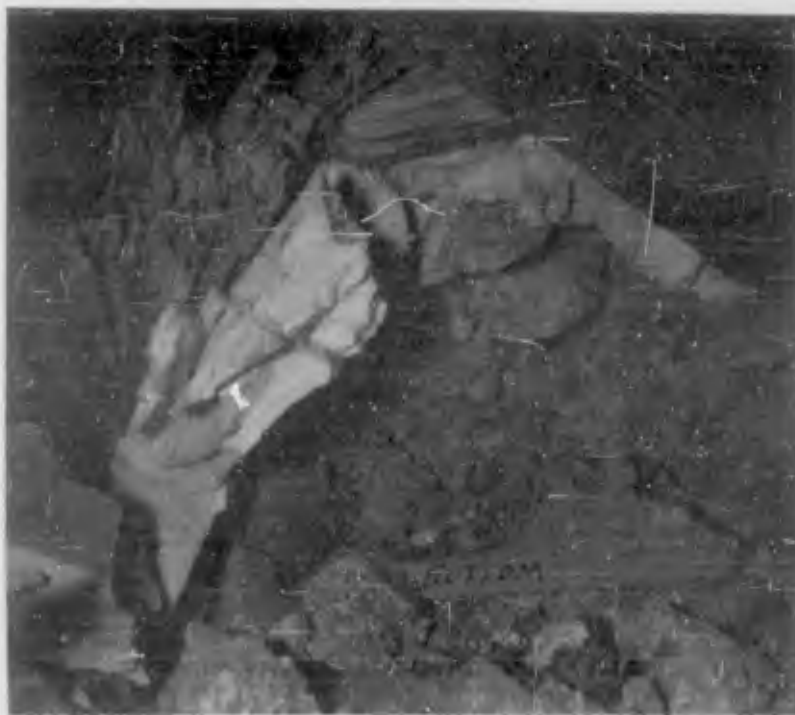
Figure 3.93 Close-up rock break through B4c (post-shot). Note broken wood lagging and compressed polyurethane foam (DASA - NOU 365-06 NTS-62).
