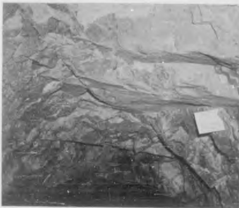
Figure 1.7 Closeup view of joints at top of tunnel. (H&N-AEC 60-762-11, 1960)
