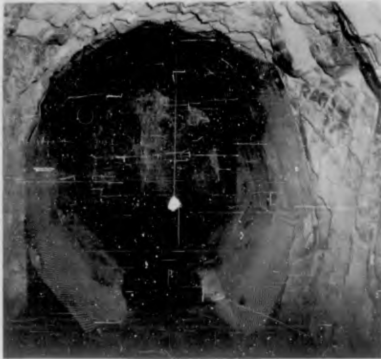
Figure 2.24 Typical installation, rock bolts and mesh, circular test section. (LRL Photo, 1960).
