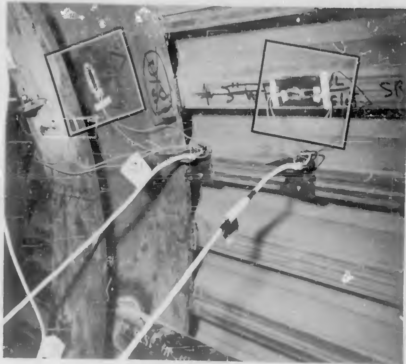
Figure 2.39 Electronic strain gages mounted to measure longitudinal strain in lining (right), and circumferential strain in wide-flange ring (left) (DASA - NOU 084-04 NTS-62).
