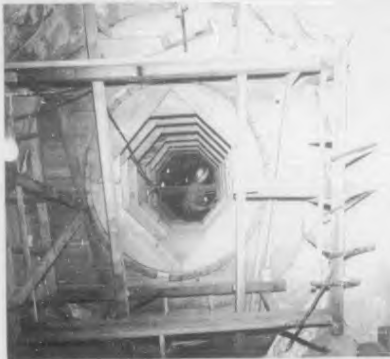
Figure 2.37 Form for concrete liner with precast foam (DASA - NOU 039-09 NTS-62).
