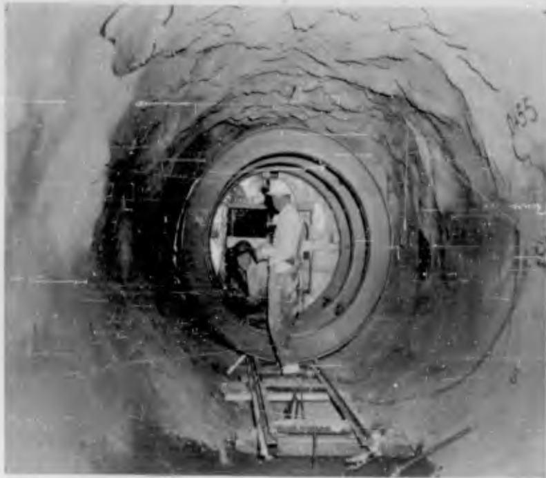
Figure 2.8 Assembling wide-flange rings on rails. (H&N-AEC 805A-5, 1960)
