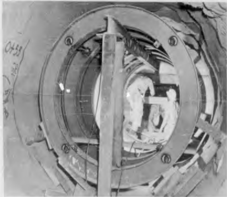
Figure 2.9 Wide-flange rings suspended on erection beam. (H&N-AEC 789-3, 1960).
