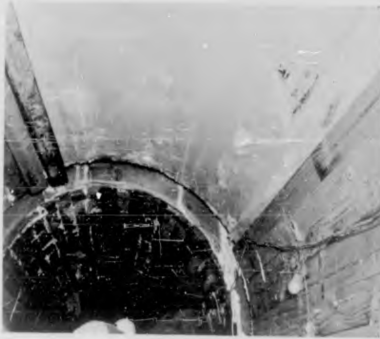
Figure 2.16 Stripping tongue-and-groove forms after foaming. (H&N-AEC 60-829-7, 1960).
