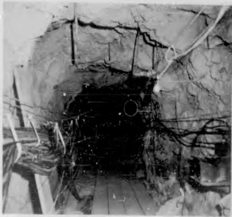
Figure 3.18 Access tunnel from Sta 4+00, approximately 410 feet from zero point, view to north (pre-shot) (DASA - NOU 085-05 NTS-62).
