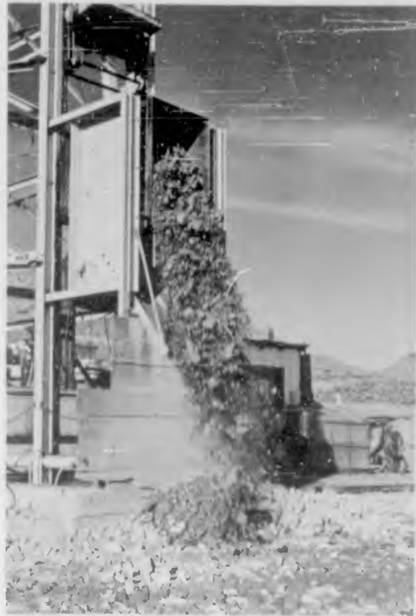
Figure 2.1 Dumping muck at Station 1500 during shaft excavation. (H&N-AEC 60-738-4, 1960).
