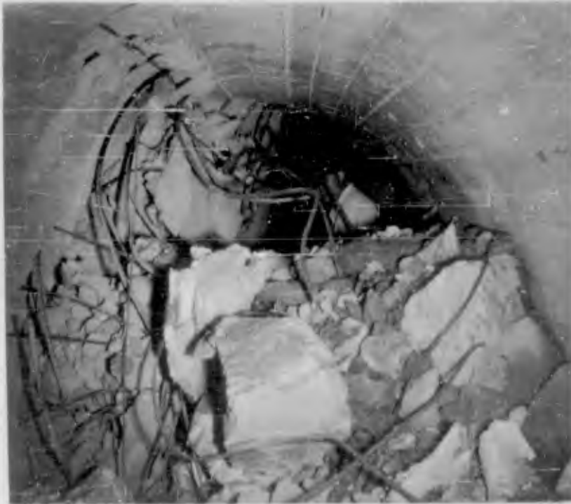
Figure 3.101 Interior view A3c (postshot), view from west. Note large pieces of polyurethane foam (white) (DASA - NOU 480-02 NTS-62).
