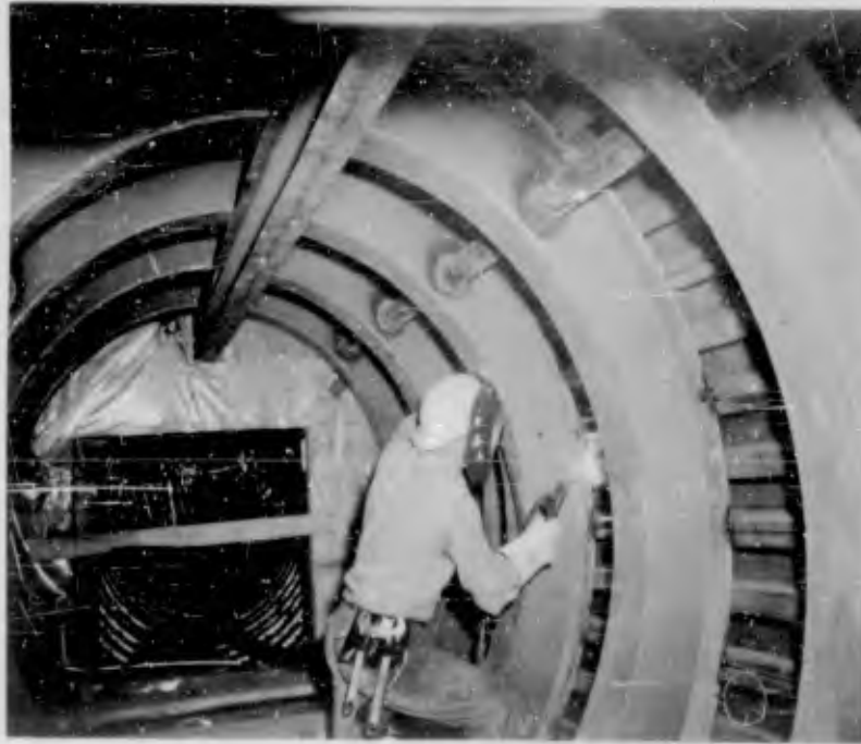
Figure 2.10 Welding corrugated steel decking to wide-flange rings. (LRL Photo, 1960).
