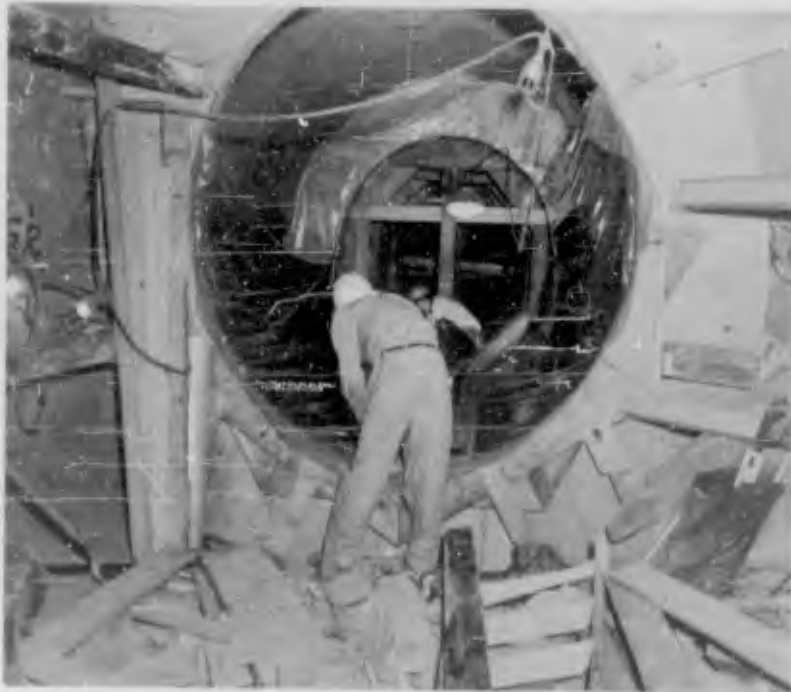
Figure 2.14 Installing polyethylene film which lined forms for polyurethane foam. (H&N-AEC 805A-1, 1960).
