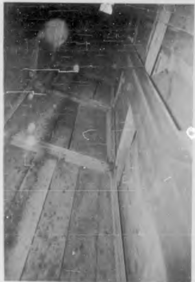
Figure 3.3 Shaft Sta 1+35, NW corner of elevator compartment. Note deformation of WF set and hanger angles. (H&N-AEC 62-1241-6, 1962).
