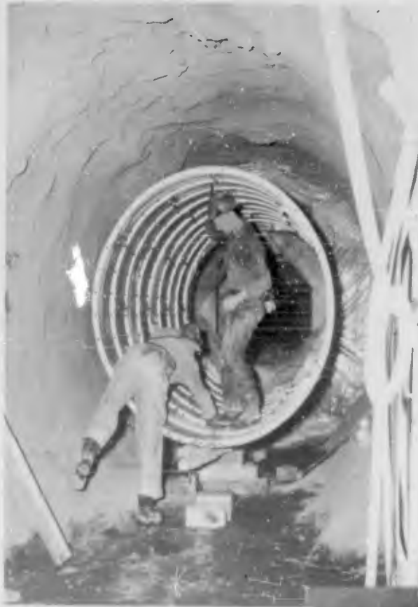
Figure 2.4 Assembling of corrugated steel tunnel liner. (H&N-AEC 792-10, 1960).
