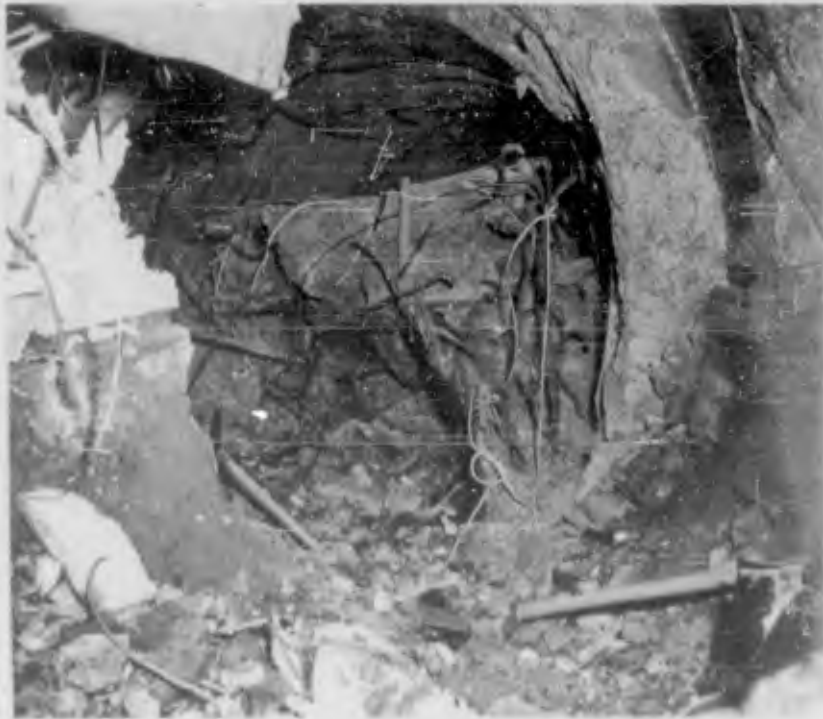
Figure 3.86 West end B3d as viewed from bypass drift (postshot). Note floor heave (DASA - NOU 339-08 NTS-62).
