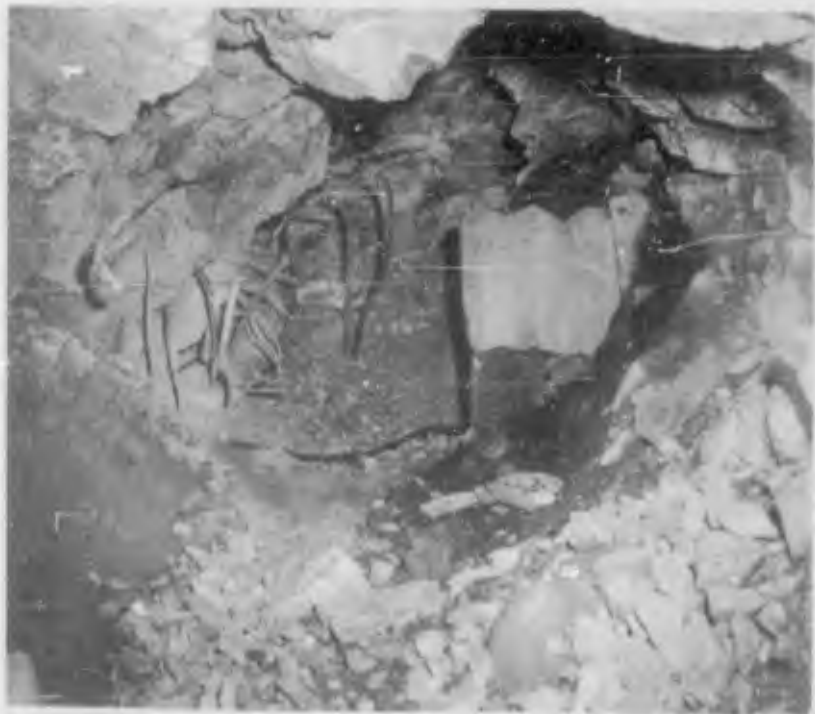
Figure 3.96 B5c (right) and B3a (left) as encountered by bypass drift (postshot) (DASA - NOU 390-09 NTS-62).
