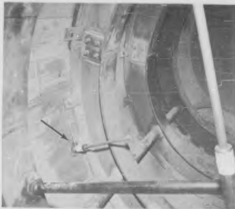
Figure 2.46 Mechanical compression-of-filler gage installed through wood lagging (DASA - NOU 070-11 NTS-62).
