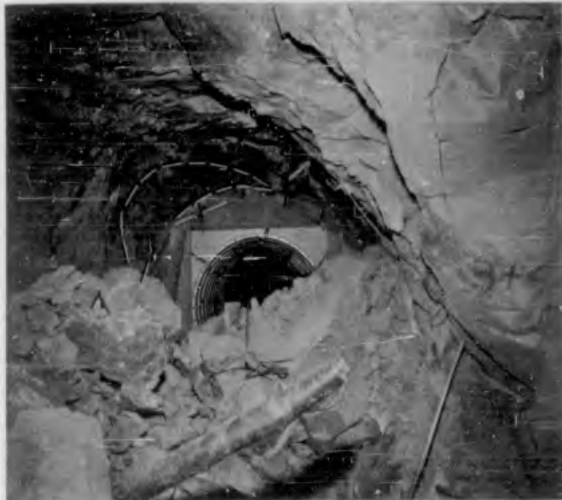
Figure 3.43 Test Section C6a and transition zone, C Drift right (postshot). Note approximate rock breakage bounded by dotted lines (DASA - NOU 206-04 NTS-62).
