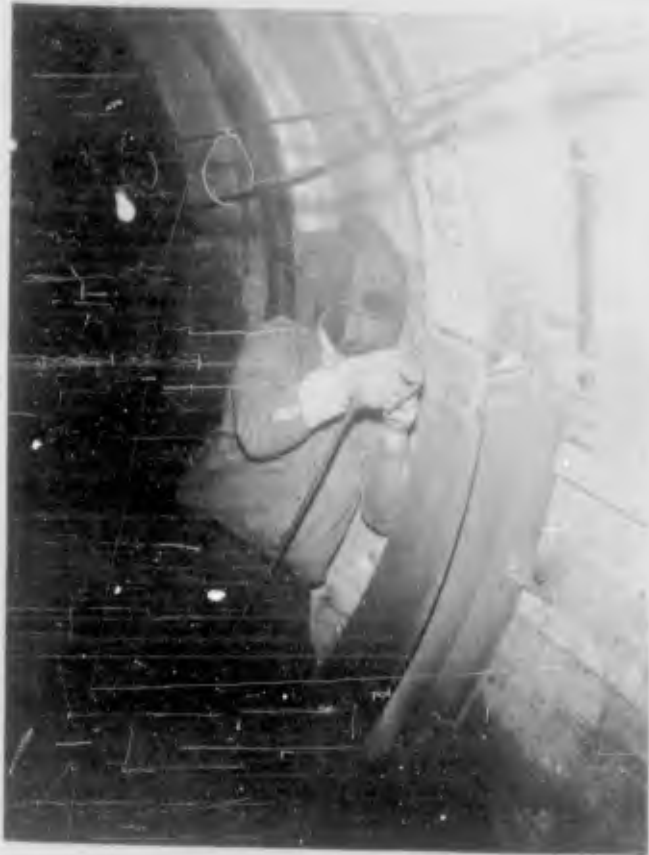
Figure 2.33 Welding wide-flange rings (DASA - NOU 044-07 NTS-62).
