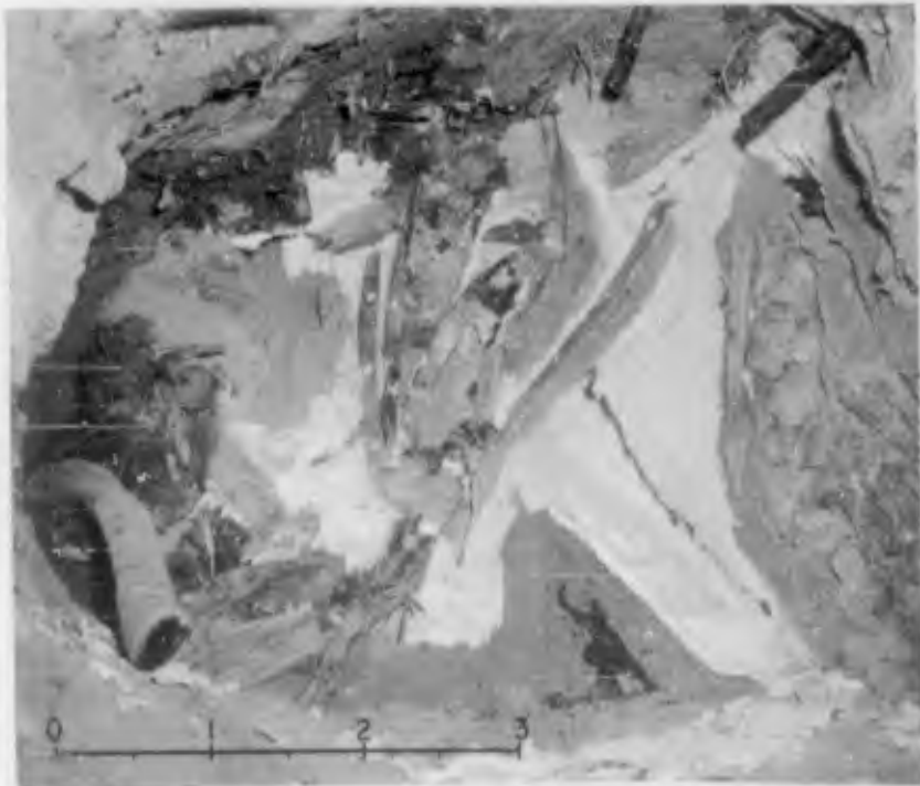
Figure 3.104 West end A5a (postshot). Note collapsed tunnel liner plates and distortion of polyurethane foam backpacking (DASA - NOU 494-02 NTS-62).
