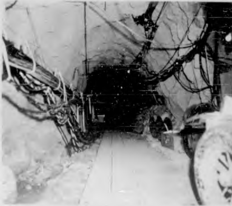
Figure 3.16 Access tunnel from Sta 3+50, approximately 460 feet from zero point, view to north (pre-shot) (DASA - NOU 085-06 NTS-62).
