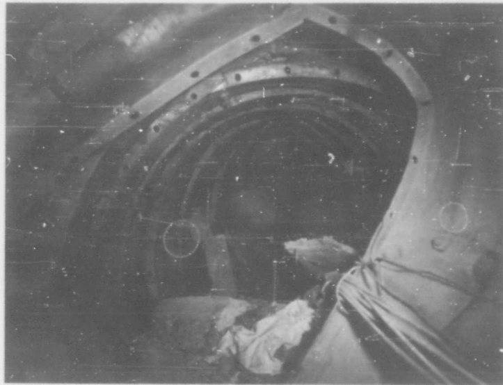
Figure 3.75 B5b from B6b (postshot). Note overlapped tunnel liner plates at the left (DASA - NOU 332-05 NTS-62).
