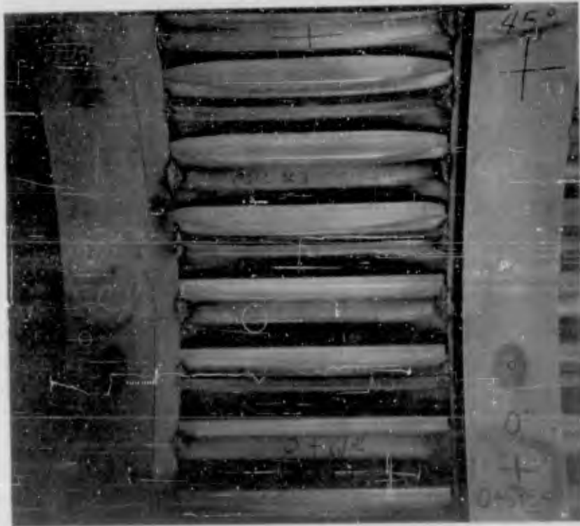
Figure 3.30 Close-up C4a. Note distorted steel decking (DASA - NOU 227-10 NTS-62).
