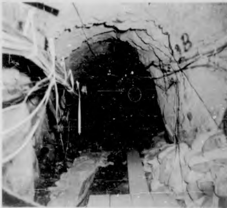
Figure 3.22 Access tunnel from Sta 5+00, approximately 310 feet from zero point, view to north (pre-shot) (DASA - NOU 084-12 NTS-62).
