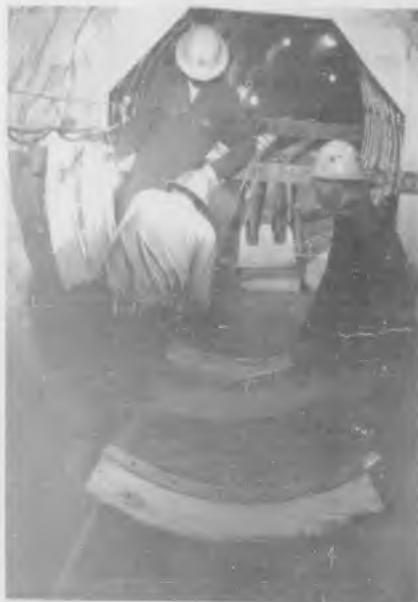
Figure 2.35 Assembling tunnel liner plates in test section (DASA - NOU 048-07 NTS-62).
