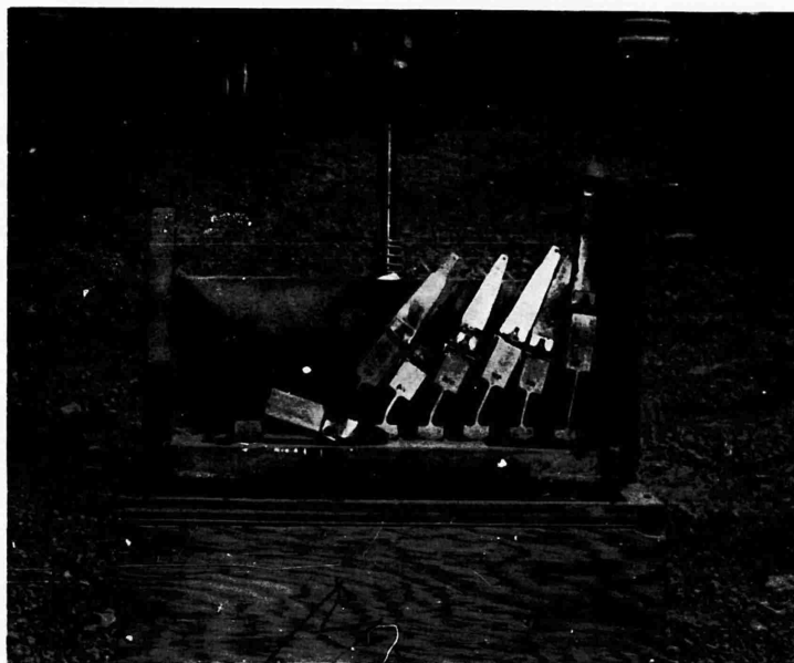
Figure 12 Additional view of damaged vertical gage from B drift access tunnel floor. (FCWT DASA 290 (NOU-238-02) NTS-62)
