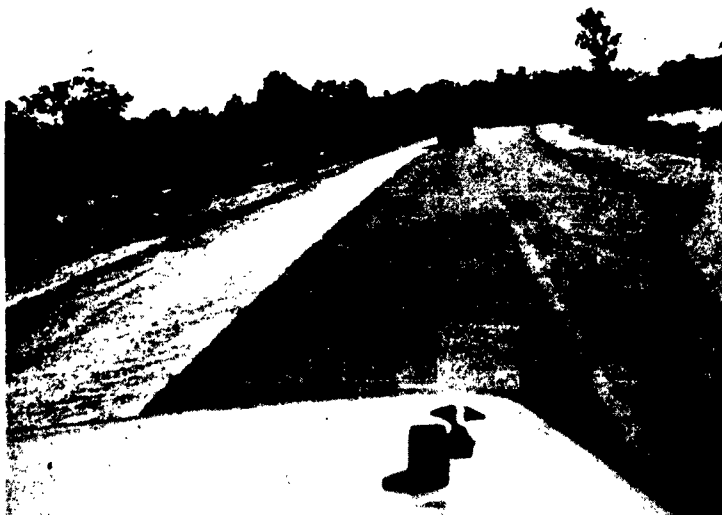
FIGURE 18. NEW PAVED HIGHWAY NORTHEAST OF KORAT
