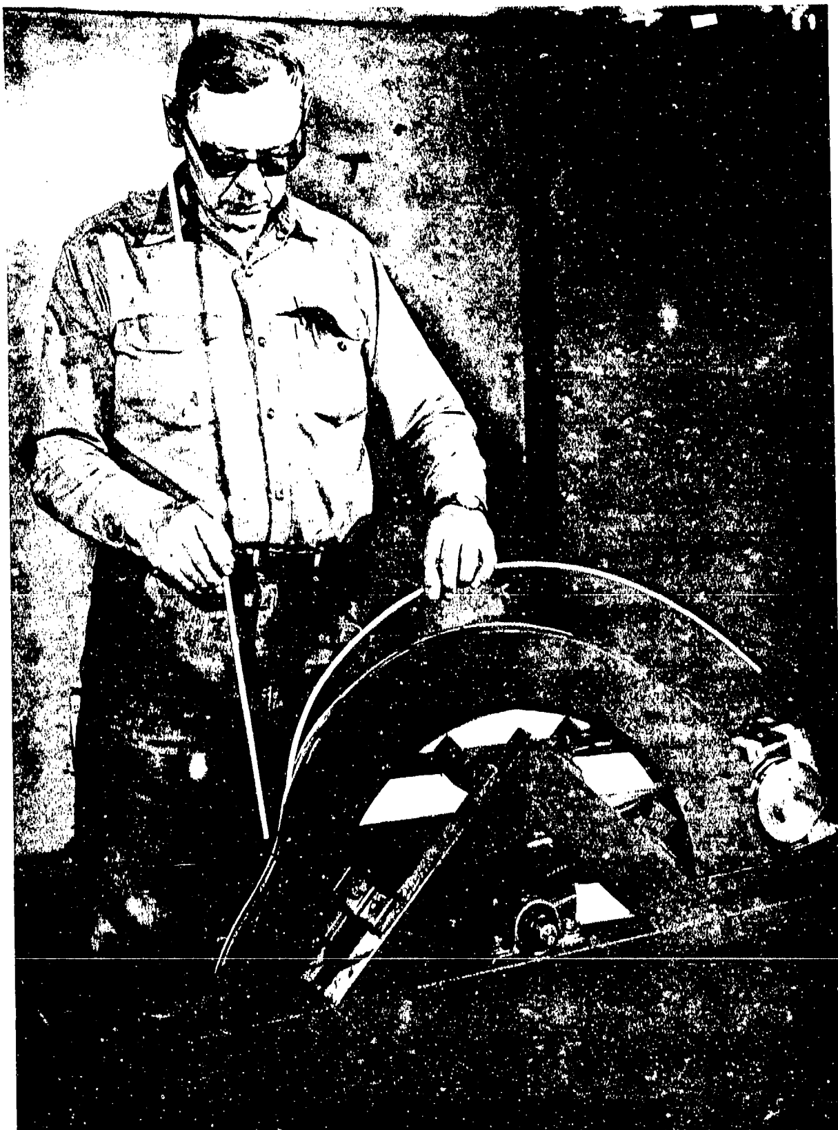
TUBE BENDING SEQUENCE
