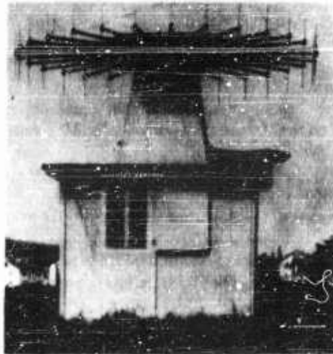
FIG. 10-51. Wide-base-line doppler direction finders for vhf range using 30 dipoles.
