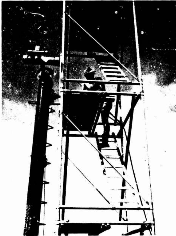
Fig. 8—Single pipe stand, showing mounting of the temperature gauge. The q-Kiel combination and the Pitot static tube are already in place.
