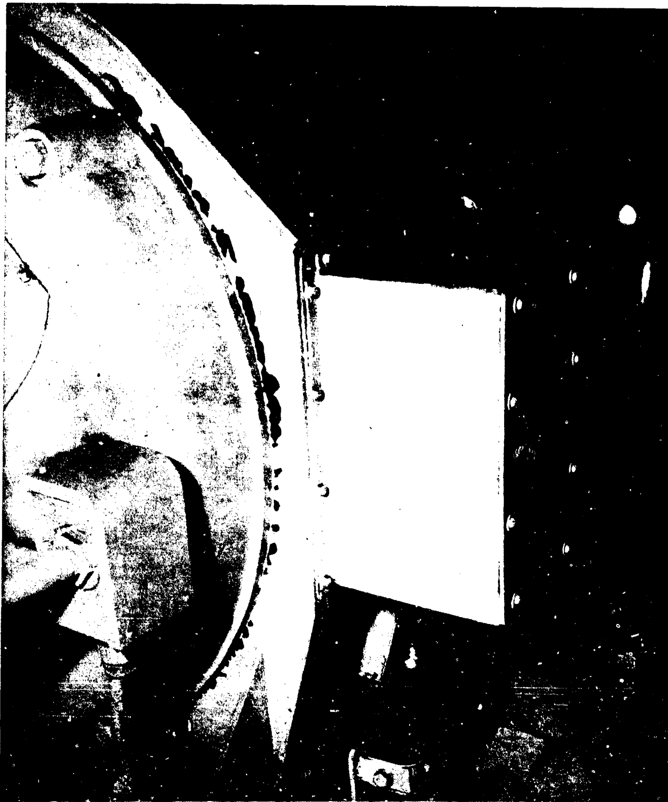
AB-CR-234-4065-3. View #3 ships service generator after engine room - looking forward. Showing cracked paint around starboard side of end bell. Evidence of heavy strain from shock.
