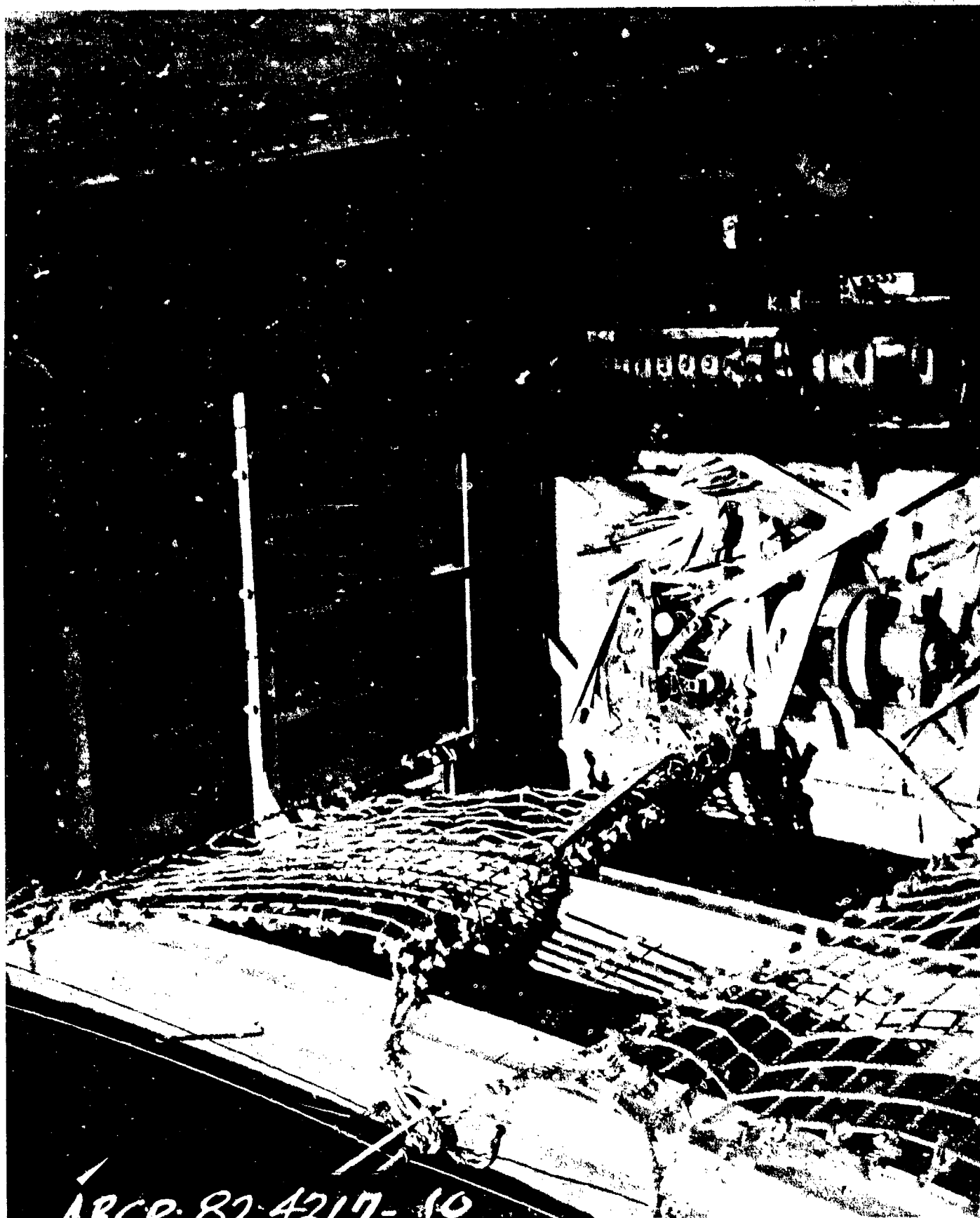
AB-CR-82-4217-10. Forward cargo hatch and damage jury rigged , cover in hold.
