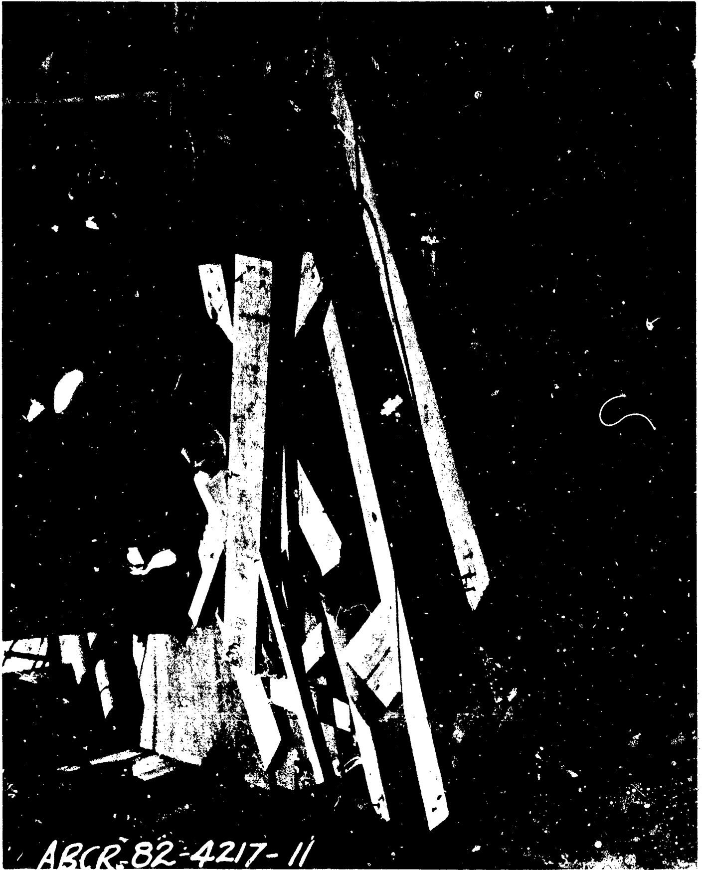
AB-CR-82-4217-11. Damaged wood cover for troop ammunition hatch, upper deck, frame 59.
