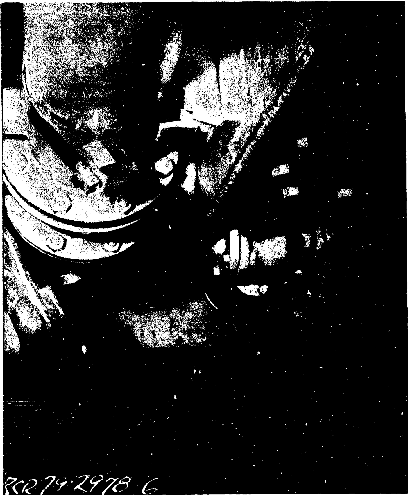
AB-CR-79-2978-6. No. 3 A.C. Auxiliary generator.
