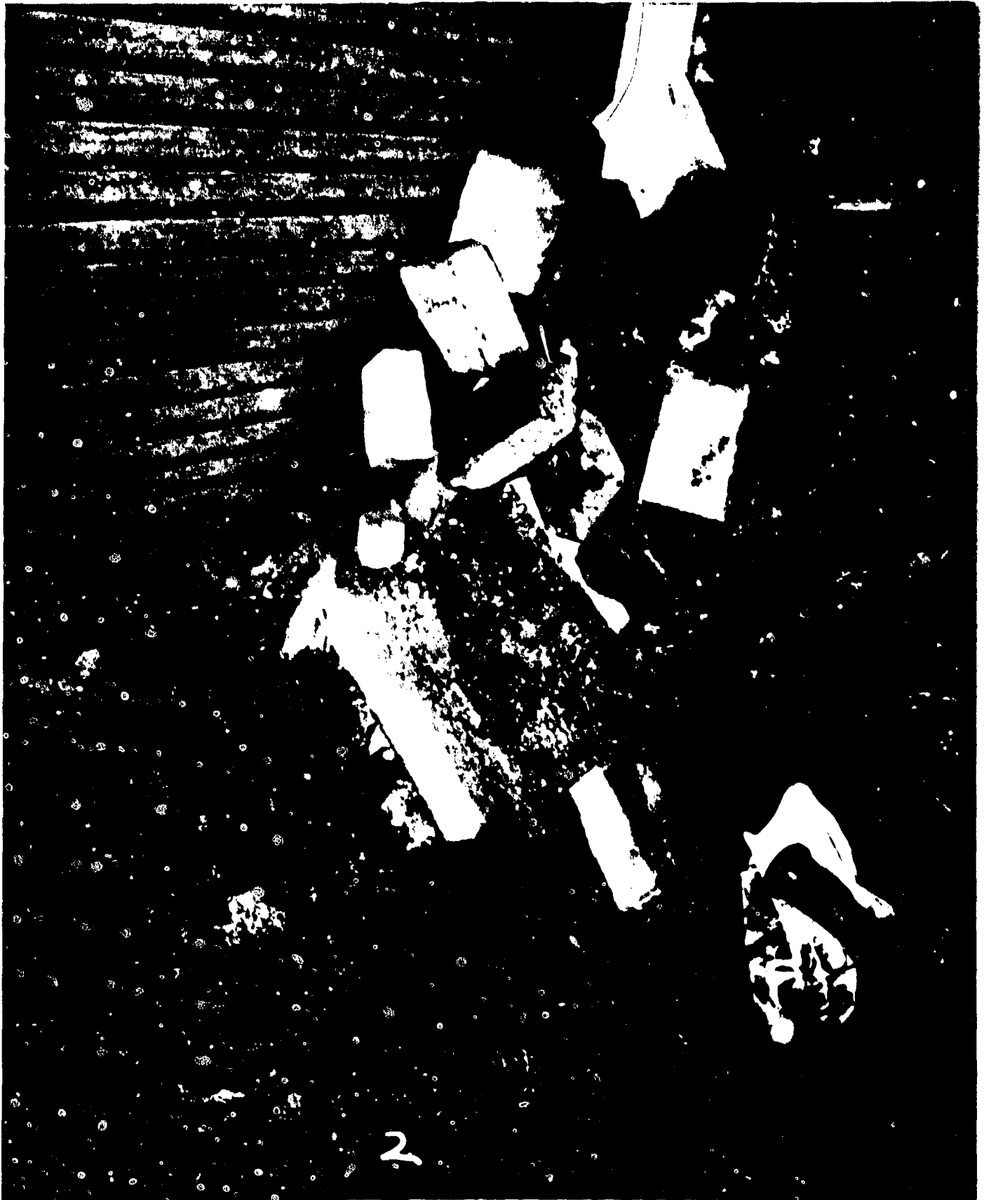
AB-CR-79-2977-2. No. 1 Boiler, dislodged floor brick.
