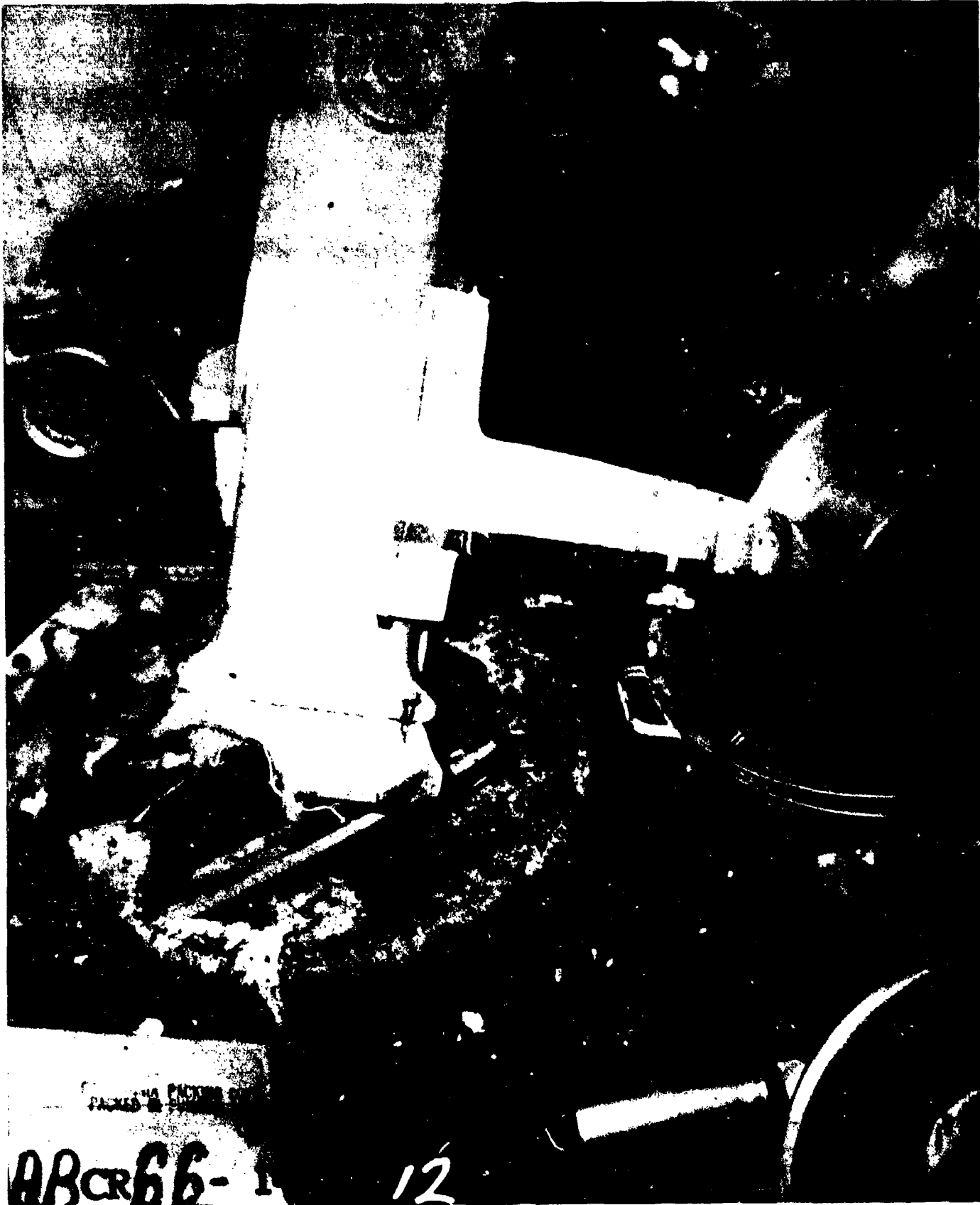
AB-CR-66-142-12. Close-up in bakery, on main deck, showing fractured dough mixer pedestal.
