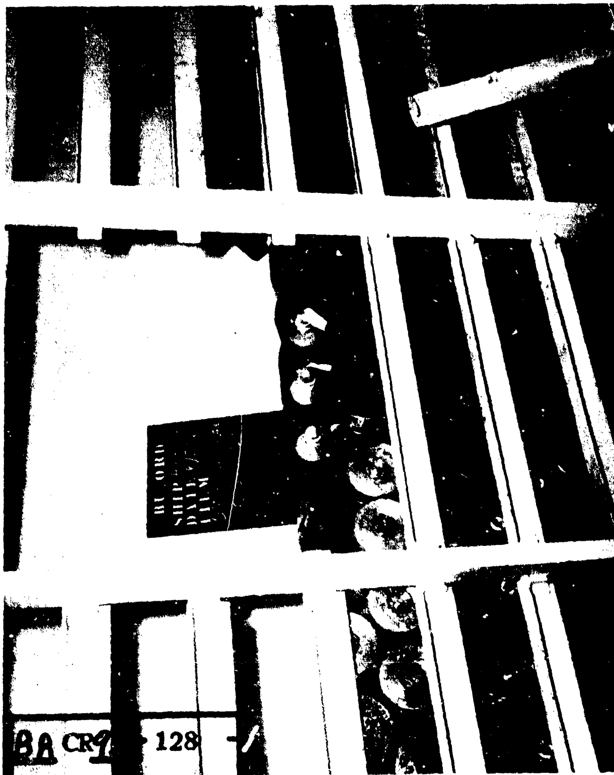
U.S.S. BARROW (APA-61) - Before Able Shows the 5".0 Aircraft Rocket Heads, plaster loaded and fused, in position prior to Test "A". The storage of Rocket Heads as shown in this view was employed for all Special Test Rocket Heads of this type. Photo. No. BA-CR-93-128-1.
